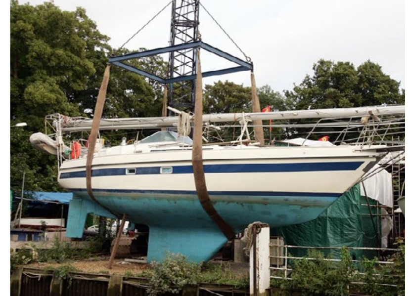
↑ Boat repair Facilities , Eel Pie Boatyard, London
