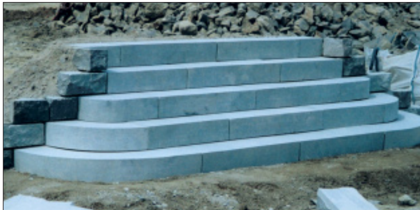
Worked ragstone for new steps pre- assembled in quarry before shipment to site
