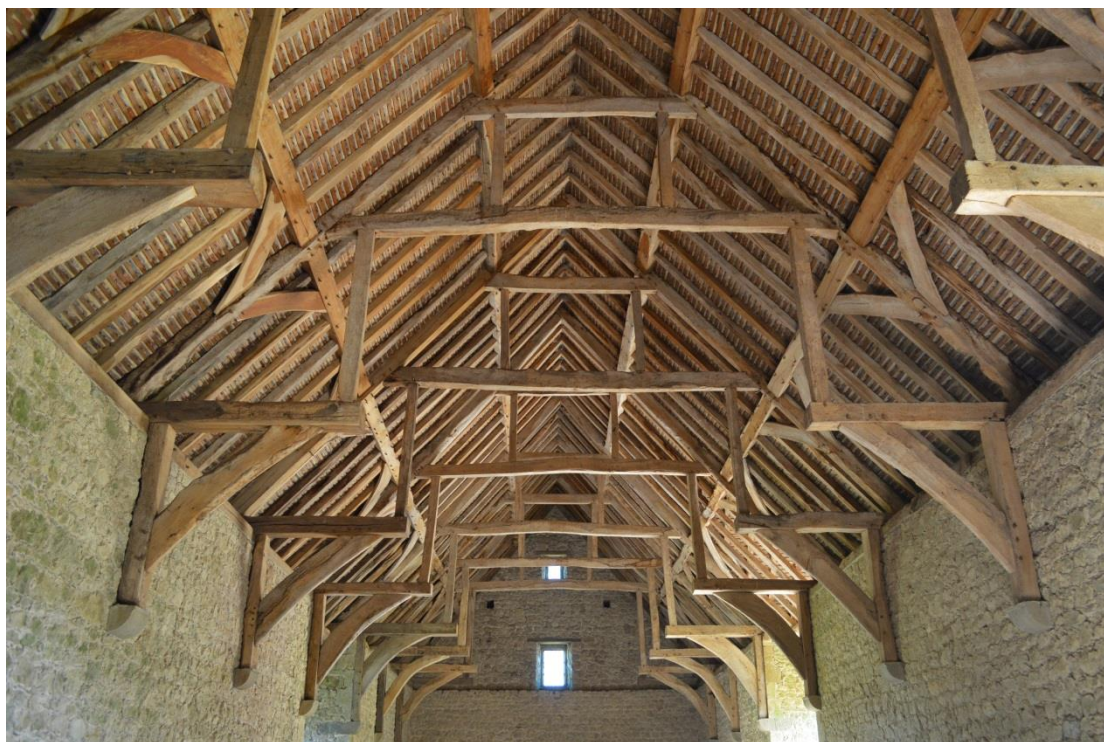
Plate 14: Westenhanger Barn – hammer beam roof
