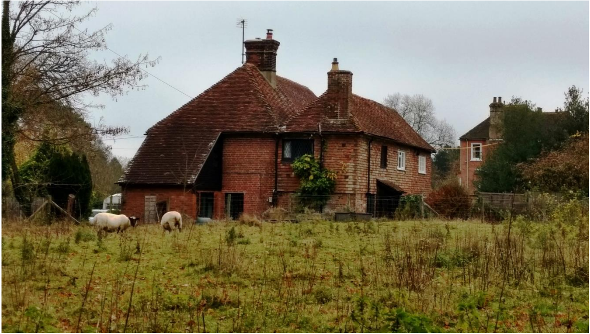
Plate 5: Old School Cottage (ADD1) – facing NE
