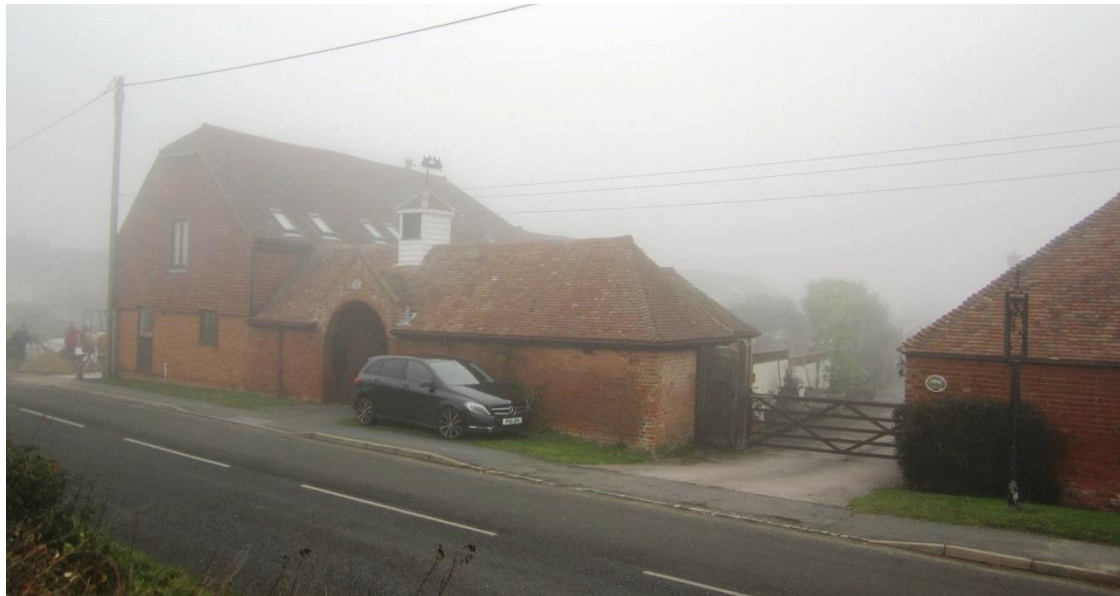
Plate 32: Newington Farmstead outbuildings – facing SW
