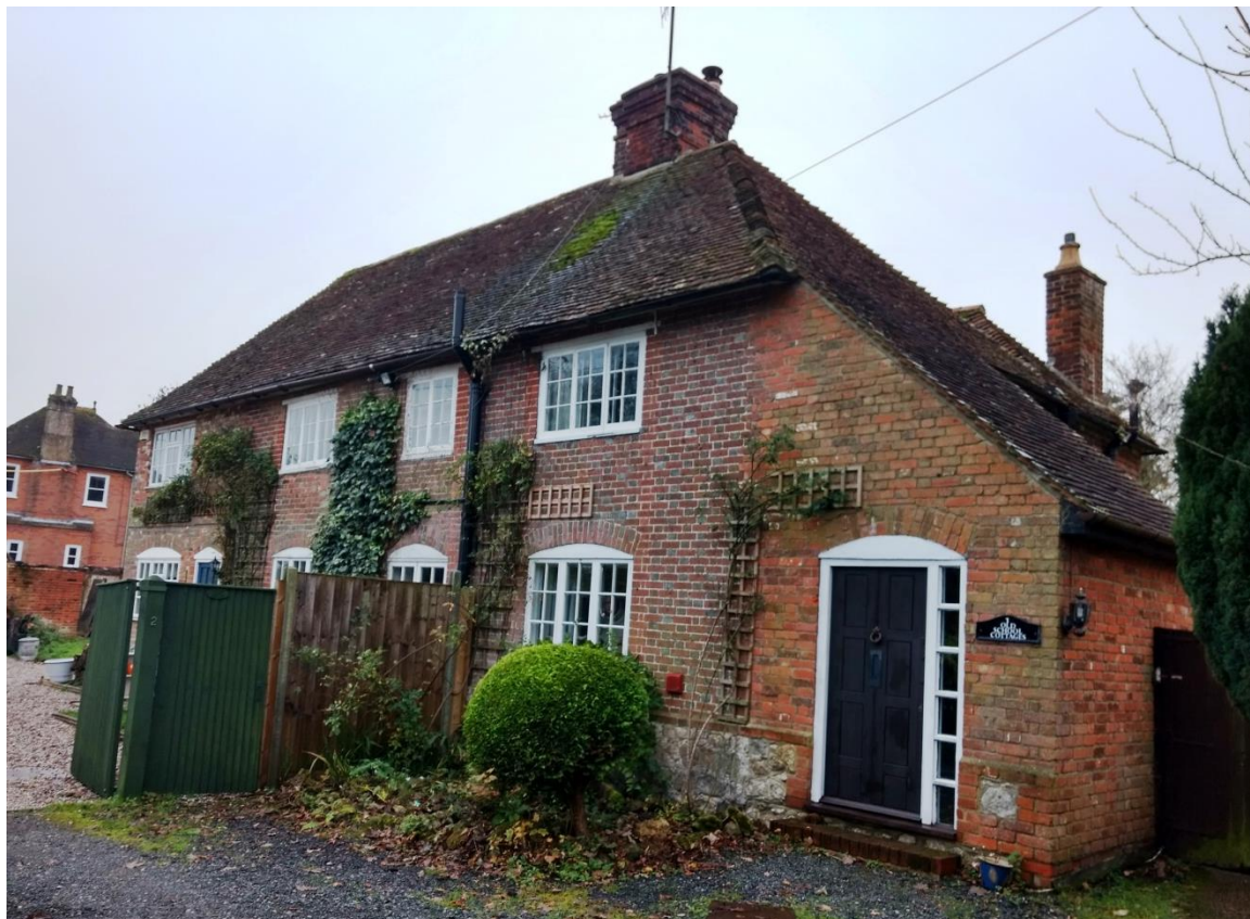
Plate 4: Old School Cottage (ADD1) – facing SE
