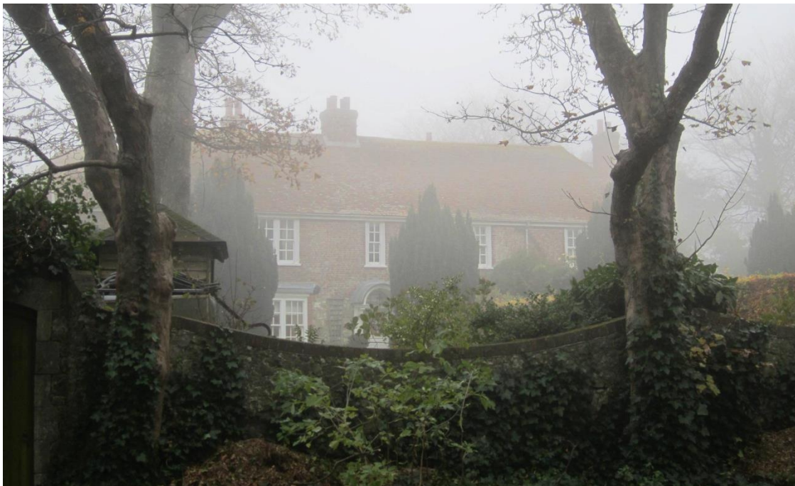
Plate 25: Bell Vue House facing N
