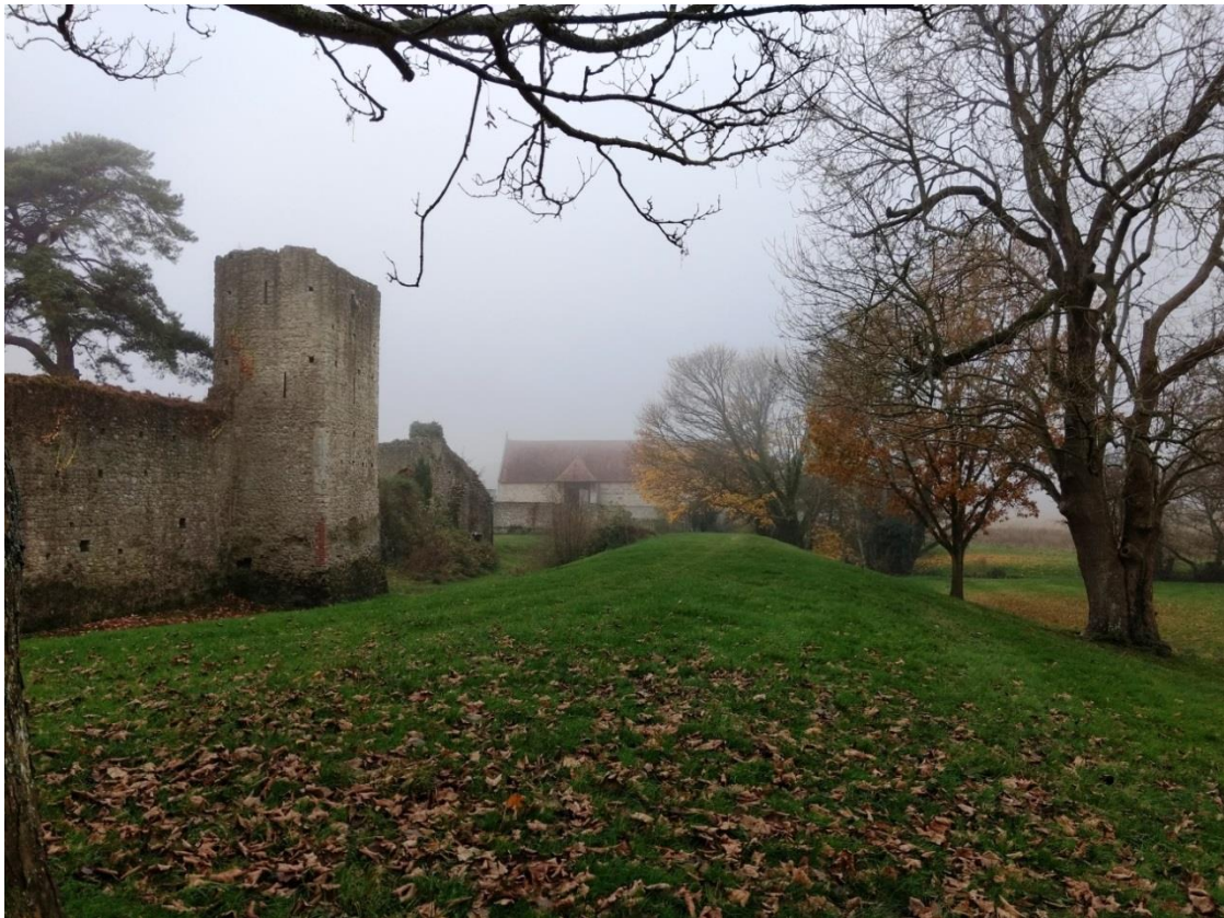
Plate 11: Westenhanger Castle (N side) and Barn – facing W
