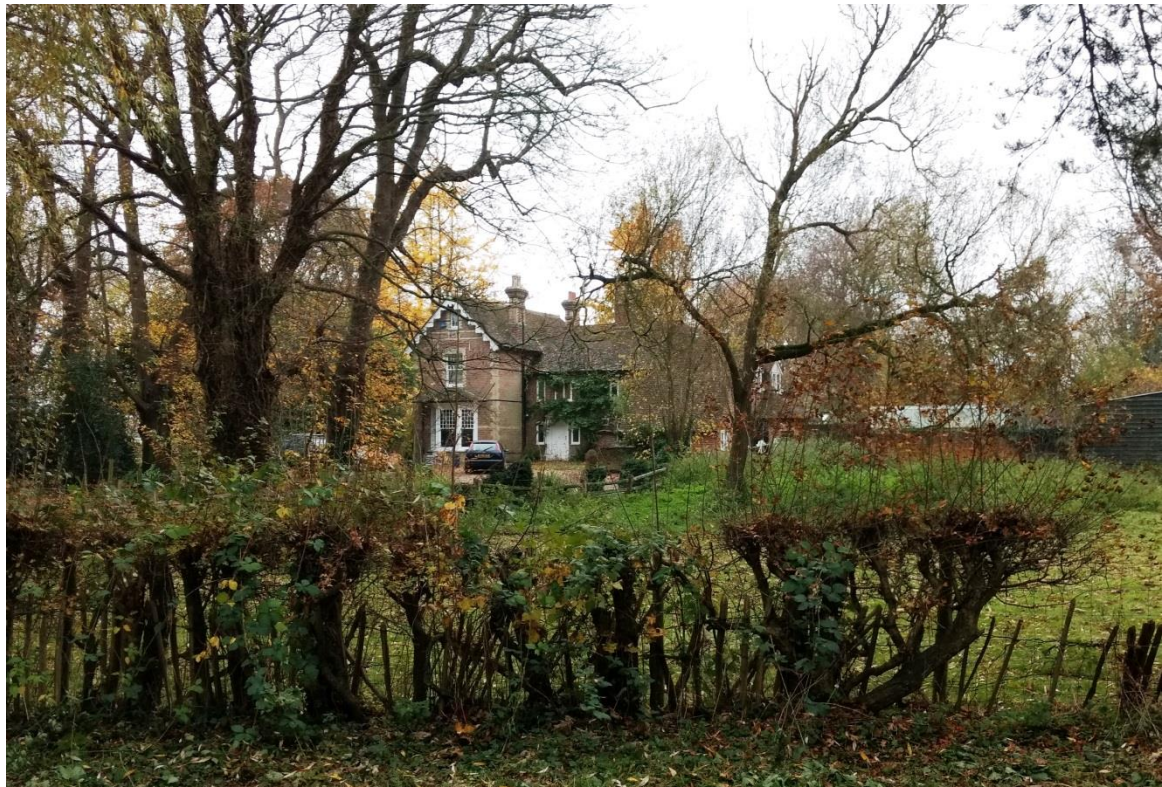
Plate 7: Grove House – facing S
