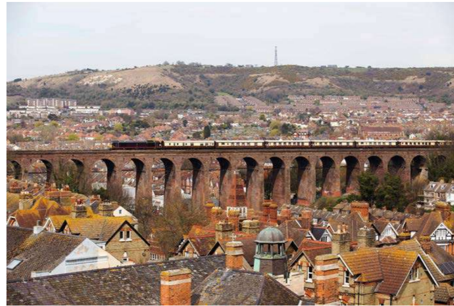
↑ Folkestone Viaduct - Foord Road Section
