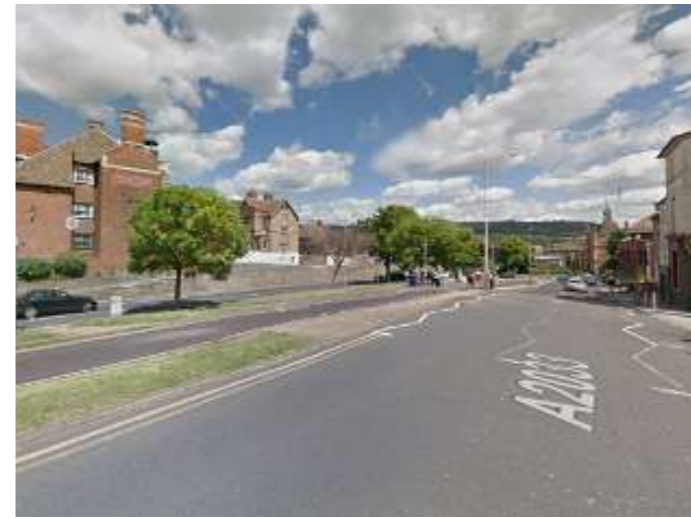
↑ Shellons Street junction with Guildhall Street: dual carriageway with multiple lanes, three-stage staggered crossing away from desire line
