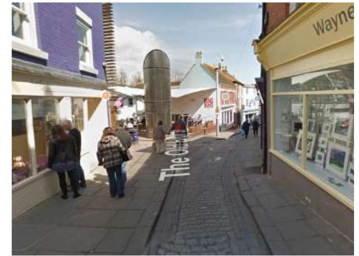
↑ The Old High Street: design treatment with kerb upstands suggests vehicles may pass through even through full-time pedestrian space (may cause pedestrians to stick to footways), cobbles are uneven, extremely narrow footway on one side
