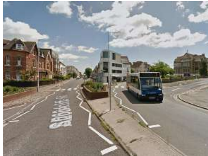
↑ Cheriton Road junction with Shorncliffe Road: wide roads, two-stage pedestrian crossing, physical barriers, and poor sense of direction to town centre
