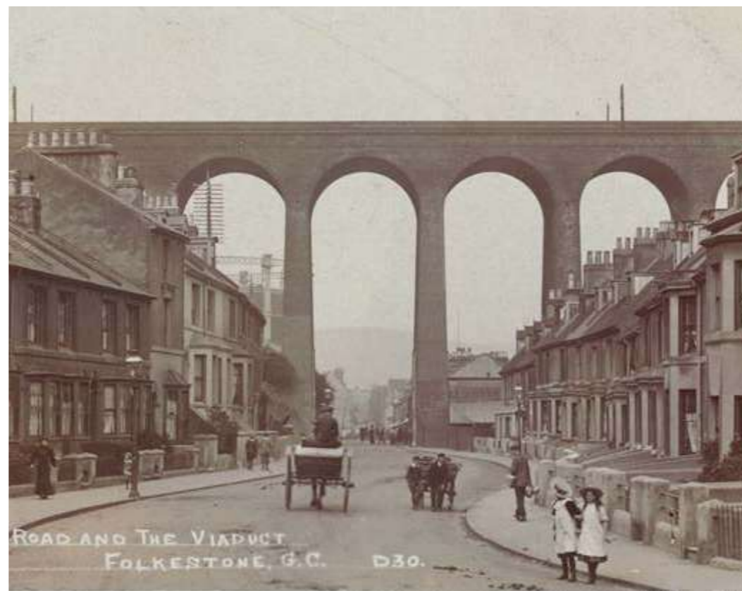
↑ 1843 - Railway Viaduct along Foord Road
