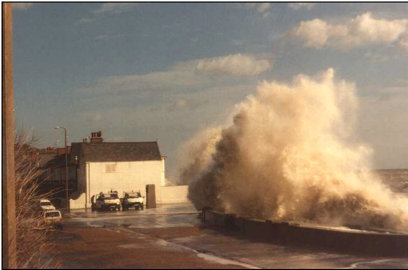
Figure 10.1 - Wave Overtopping at Sandgate, December 2000
