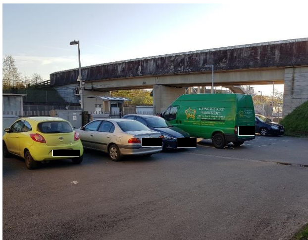
Photograph 13 Westenhanger Station Car Park
