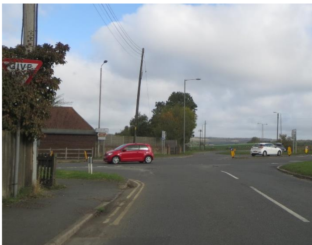
Photograph 11 Stone Street South-bound, approaching Aldington Road
