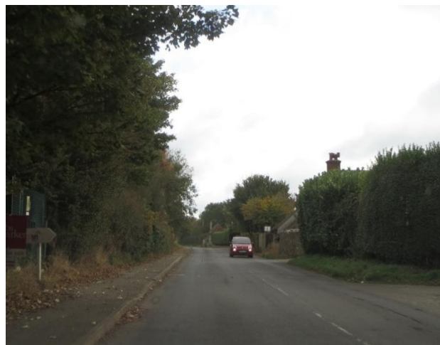
Photograph 10 Aldington Road West-bound
