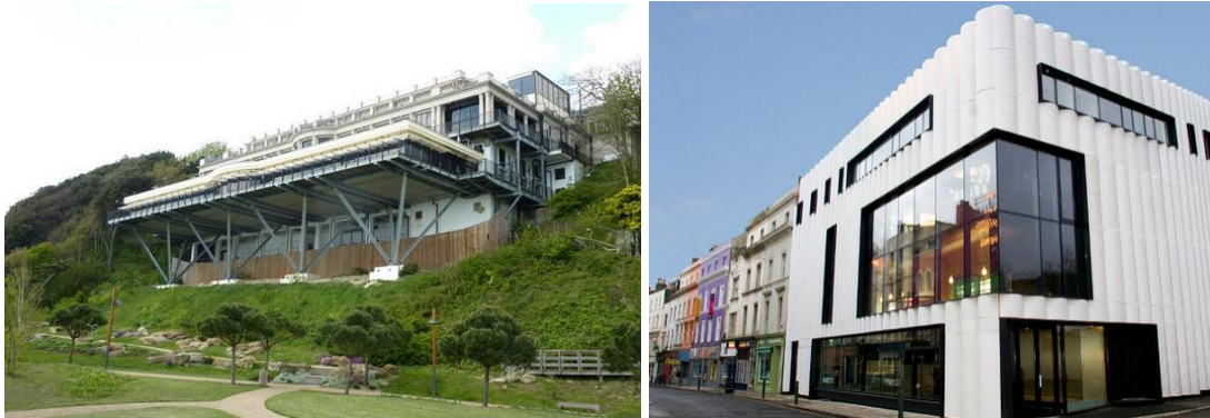
Figure 7.1 - Leas Cliff Hall and Folkestone Quarterhouse
