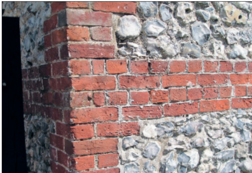
Right: Flint walling with brick quoins
