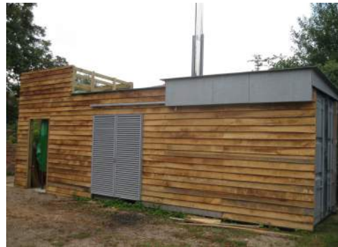
Oak clad woodfuel boiler
