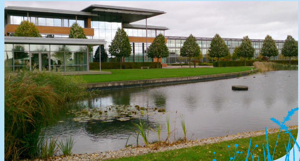
Cambourne Business Park © 2016
