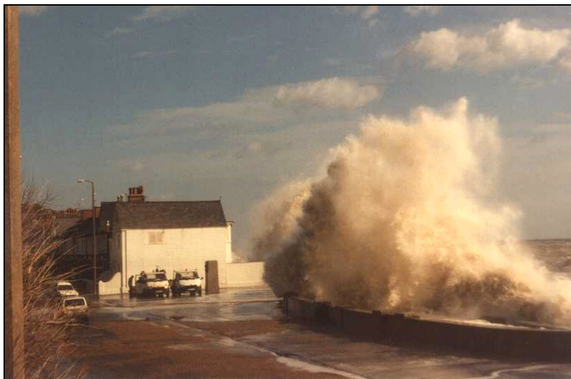
Figure 10.1 - Wave Overtopping at Sandgate, December 2000
