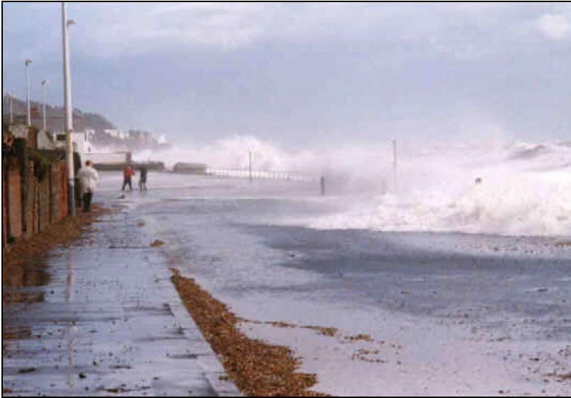
Figure 6.1 – Wave overtopping along Sandgate Esplanade, 24 October 1999
