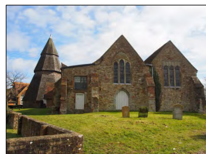
Fig. 45: Brookland church, with its distinctive detached shingle steeple
