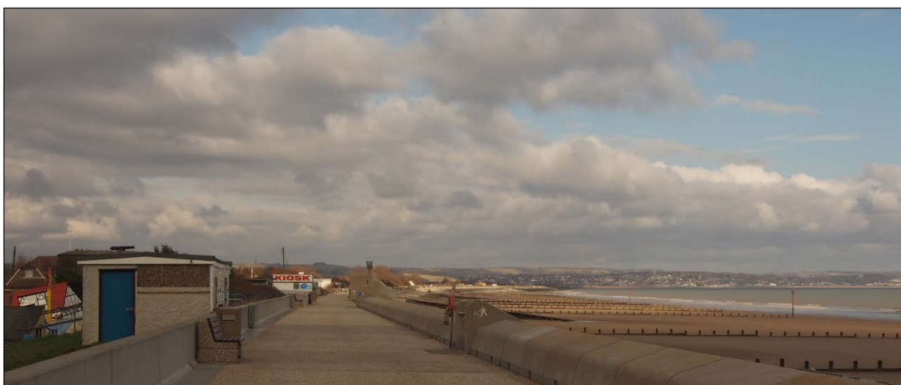
Fig. 63: The Dymchurch wall looking north. Note the cannon mounted on the Martello tower on the left.
