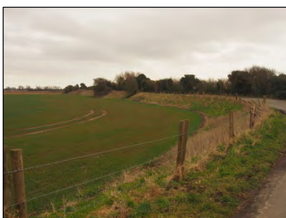
Fig. 44: Elevated lane along the Hook Wall, a medieval sea wall at the southern boundary of the LCA
