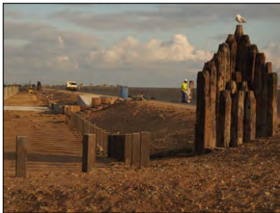
Fig. 35: Sea wall repairs near Camber
