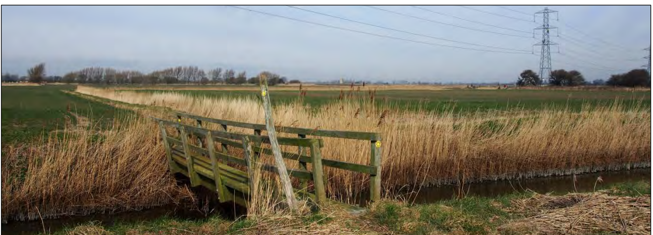
Fig. 46: Bridge over Tore Petty Sewer, near Midley Church
