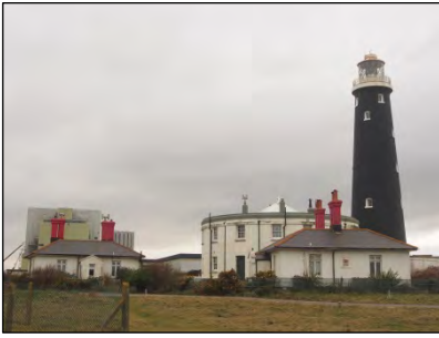
Fig. 23: 1904 lighthouse and earlier cottages, Dungeness. The power station is visible beyond
