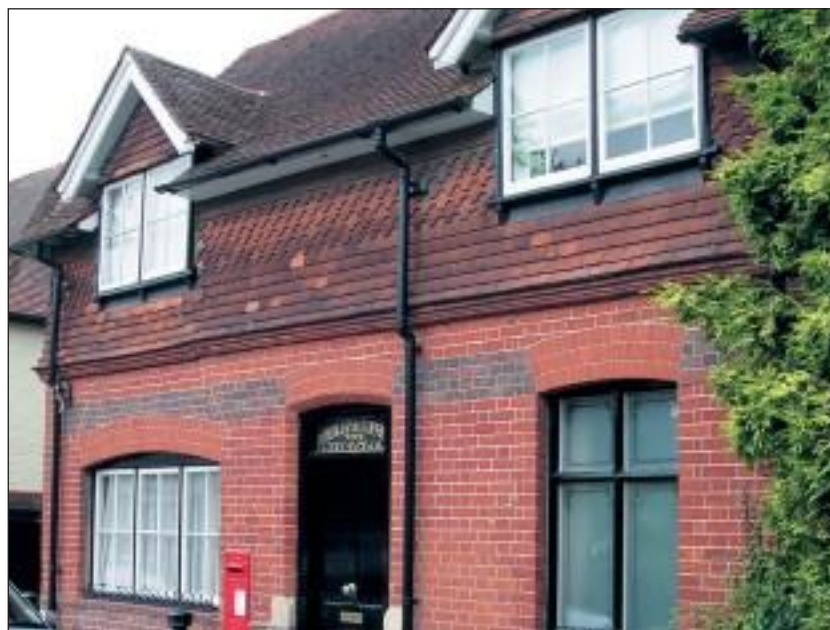
Tile hanging on upper elevation of traditional brick building
