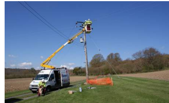
Removing overhead cables
