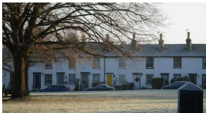
Houses at Bessels Green
