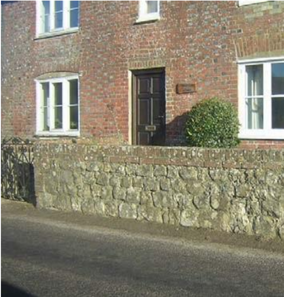
Brick and ragstone wall and cottage in Lympne
