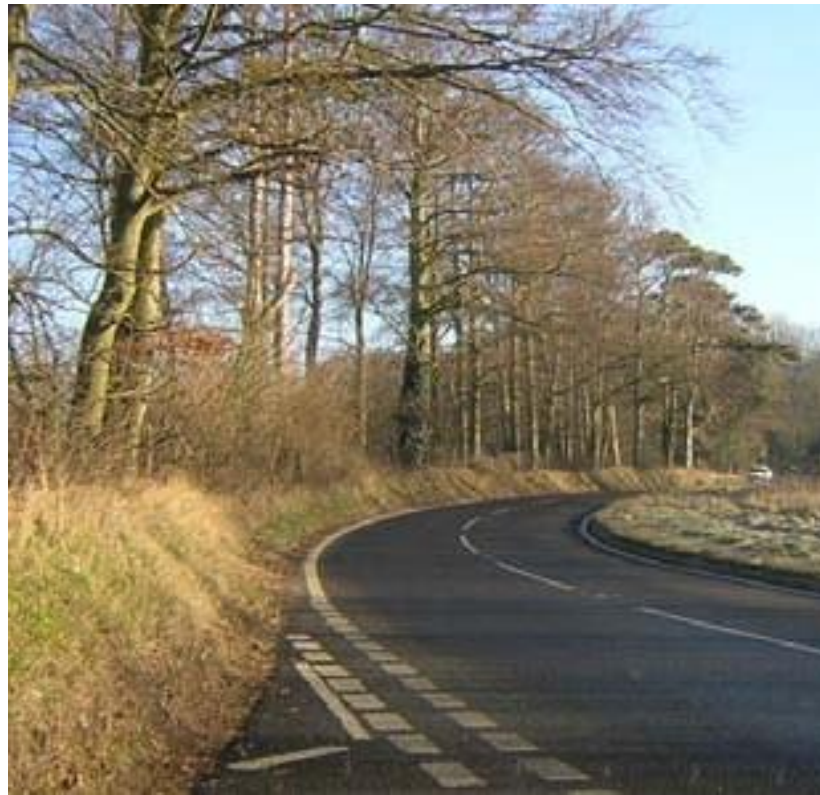
New road alignments detract from historic character
