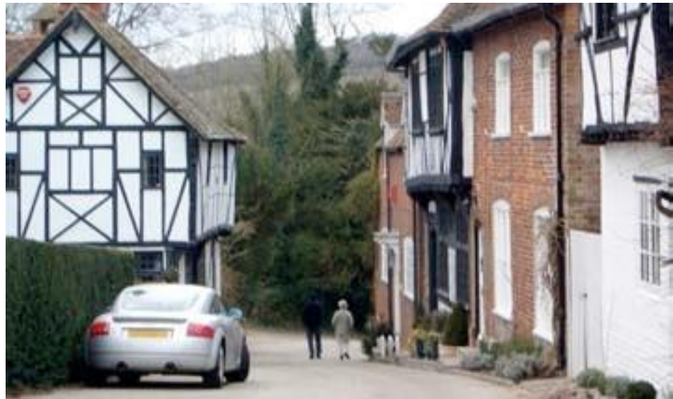
The streetscape as an integral part of the built environment (Chilham)
