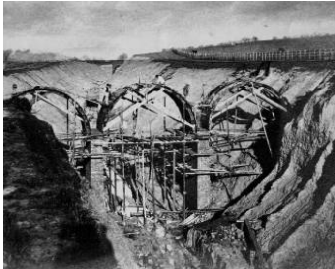
Building the railway cutting
