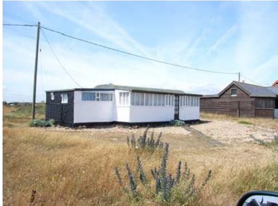
Railway carriage converted into what have now become permanent homes
