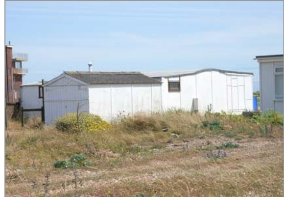
The evolution from railway carriage to a more permanent dwelling is still evident
