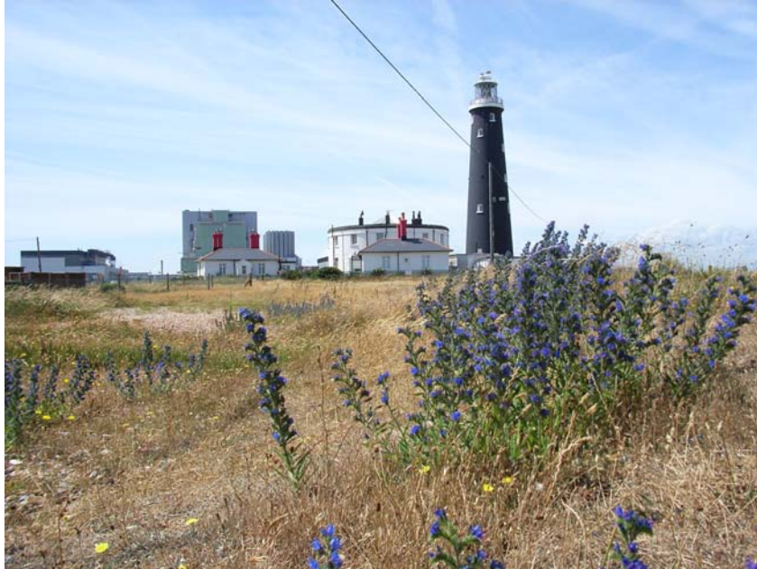
View of Dungeness power station and lighthouse
