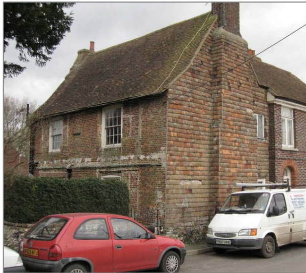
Water Farm, with blocked cross windows visible on main front
