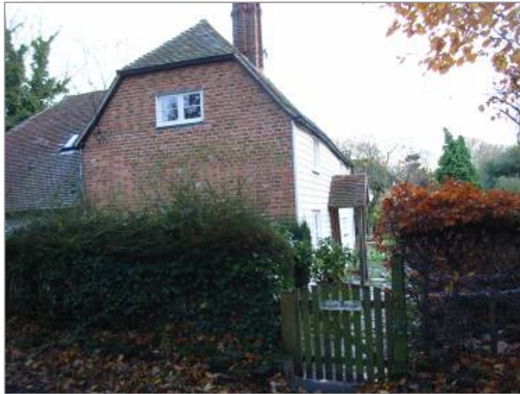
Above: Magpie Cottage shows gable end with mathematical tiling; Below: Old Kent Cottage
