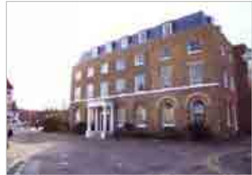
The Mackeson Offices, 1 The High Street
