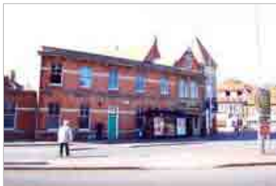
This building, which forms the corner of Prospect Road and the High Street, has good form but requires conservation and enhancement to add value to its prominent location
