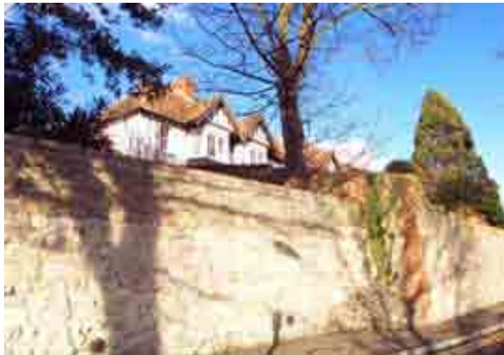
Edwardian houses sit on high ground above medieval retaining wall
