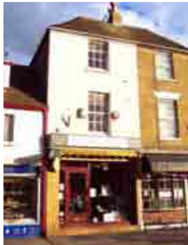
A poorly designed shopfront, out of keeping with the scale and proportions of the parent building
