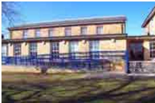
The 1930's Oaklands Library building
