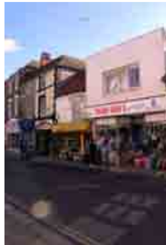
Shopfront façade out of keeping with the High Street
