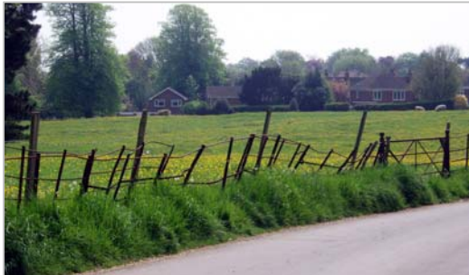
Railings in Boundary Lane need maintenance
