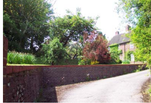
The new boundary wall at Benover House has used local materials and detail
