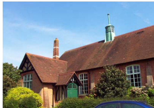
Village Hall from Rectory Lane
