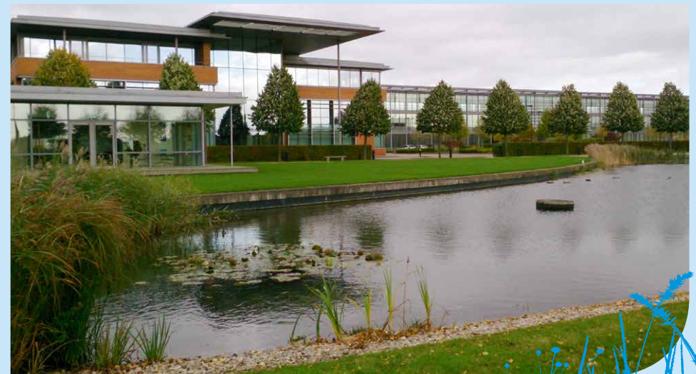
Cambourne Business Park © 2016
