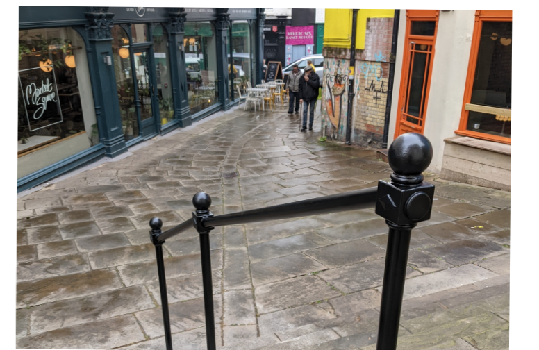
Repointing of the pavement and new handrails installed off Rendezvous Street, Folkestone as part of public realm improvements funded by the 'Welcome Back Fund' during the year.
