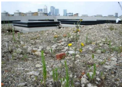
Photograph 44: Example of green roof black redstart (Photograph obtained from Black redstart roof three years after construction (photo by D. Gedge). | Download Scientific Diagram (researchgate.net))
