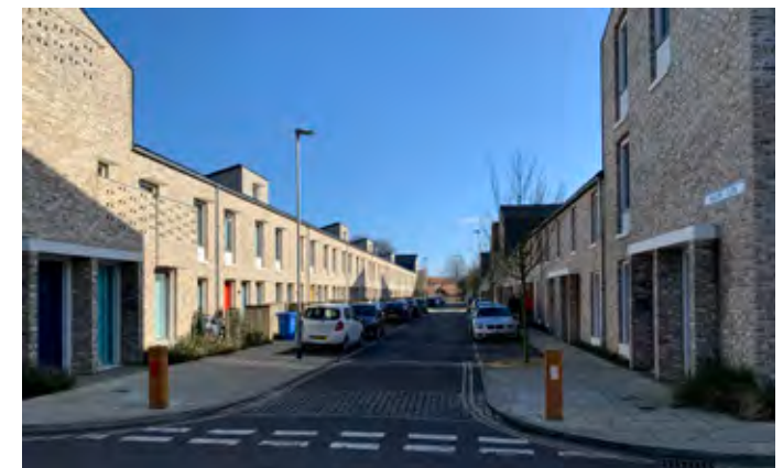
Fig. 5.43: Consistent character in the main terrace at Goldsmith Street, Norwich, with the corners introducing a low-key 'landmark' moment with slightly taller building volumes.
