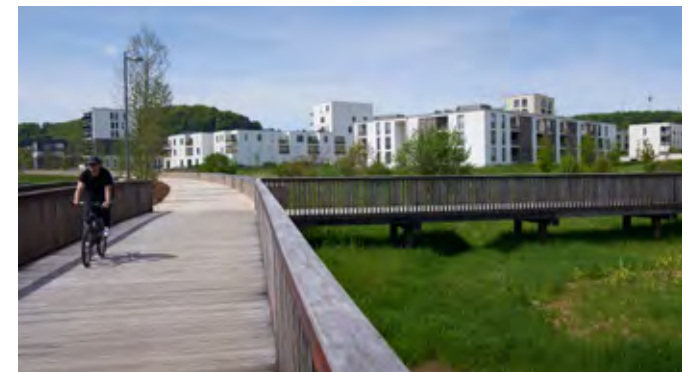
Fig. 5.6: Elevated pathways positioned over a softly landscaped attenuation basin provide routes between destinations
