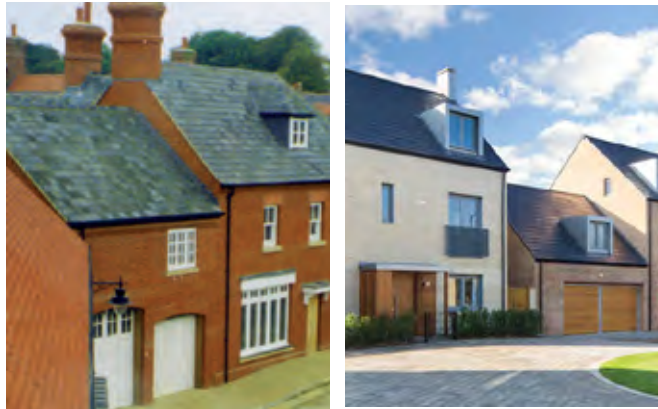
Fig. 5.54: If they are thoughtfully located and carefully designed, garages can make a positive contribution to the street scene
