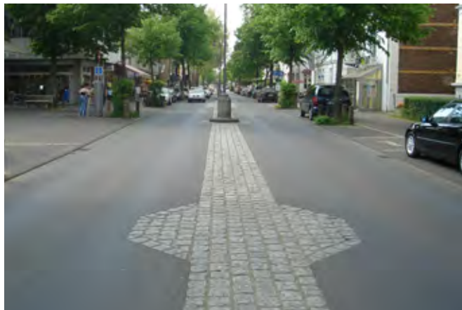
Fig. 5.30: Median strips in different materials can help to visually narrow the carriageway, slowing traffic and creating a more people-oriented environment in urban areas
