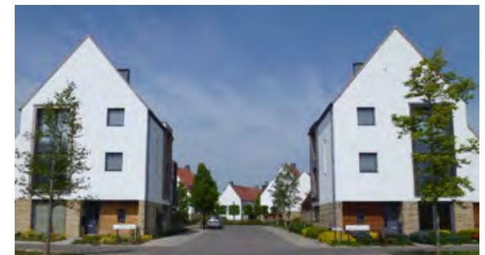
Fig. 5.12: Gateways may be local in character: here at Derwenthorpe the two strong gable ends create a memorable approach to this cluster of homes
