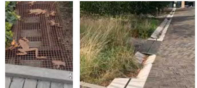
Fig. 5.5: Urban SUDS features (e.g. swales and rills) provide water management and playful features within public open space (left - Stockholm, Sweden, right - Cambridge)
