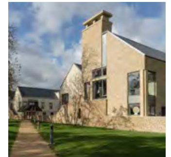
Fig. 5.40: This building maintains the privacy of the ground floor whilst also providing active overlooking of the green space.
