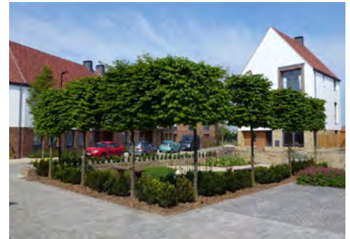
Fig. 5.53: A resilient approach to parking: the public realm works with and without cars
