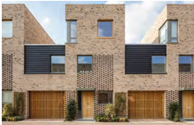
Fig. 5.56: Carefully designed integral garages work with the overall building design, whilst overlooking of the street is provided from upper floor windows - a solution that should be avoided for long stretches as the frontage is not sufficiently 'active'
