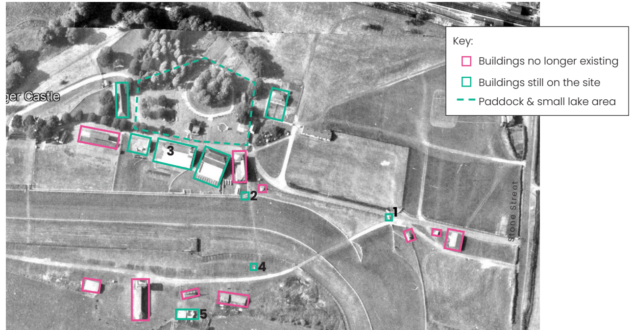
1960s photograph of Folkestone Racecourse, identifying remaining and removed buildings
