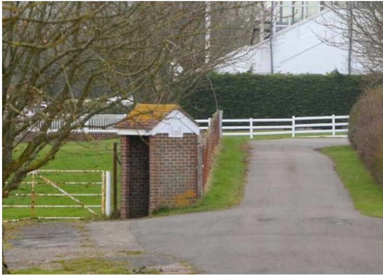
Small brick watch building (1). (Note: numbers in these photos refer to the key plan on p33, and are not heritage asset numbers)
