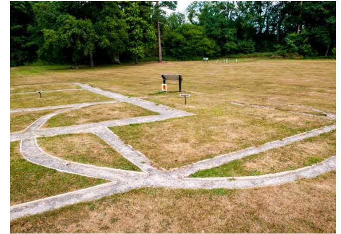
Rockbourne Roman Villa, Hampshire where the layout of the First House buried below is made manifest in the ground surfaces.
