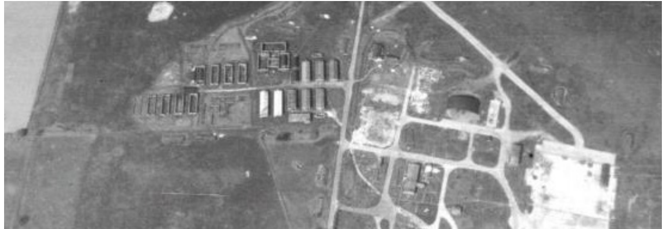
Structures either under construction or partially demolished shown on the 1940s aerial photography
