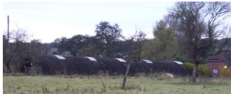
Former munitions store and extant Nissen Hut (WS20)
