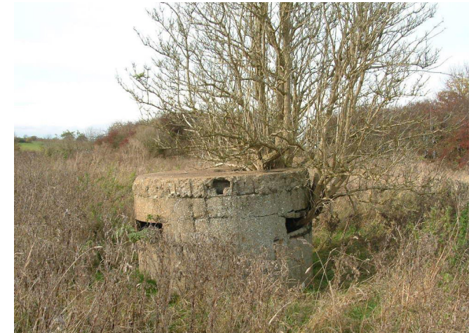
Pickett Hamilton Fort (32). Note: this is outside the application boundary but within the wider framework masterplan area.
