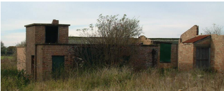
Gas decontamination building (30). Note: this is outside the application boundary but within the wider framework masterplan area.
