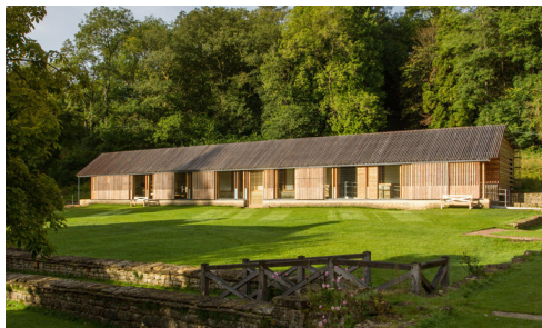
Chedworth larch-clad shelter over Roman ruins
