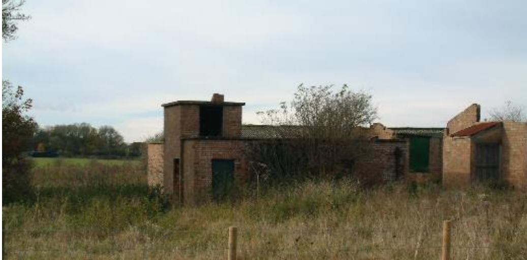
Plate 24: Gas Decontamination Building, Otterpool Lane (30)
