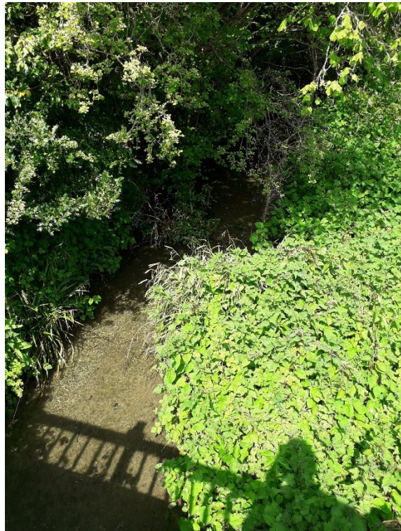
Photograph 23: Bridge crossing over water body 32 in 2020 survey
