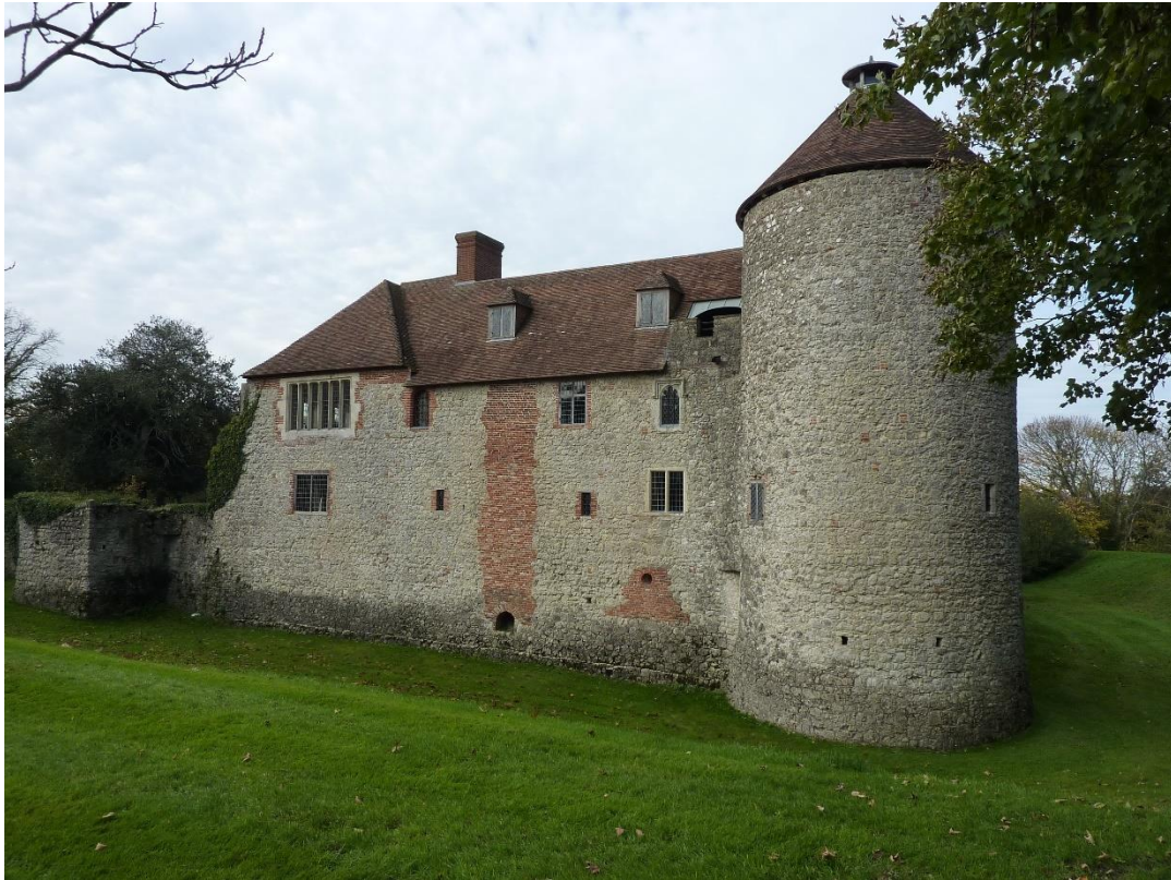
Figure 4. View to the east range of the castle and the dovecote tower (the OS's annotation of this as 'Fair Rosamund's Tower' is misplaced) from the possible terrace walk. The continuation of the walk along the north side of the castle can be seen to the right.
