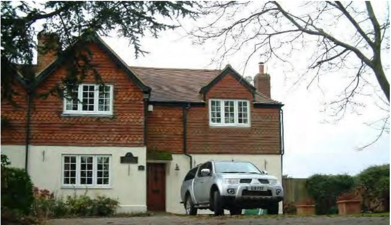
Plate 15: Cottages to the west of Harringe Court.
