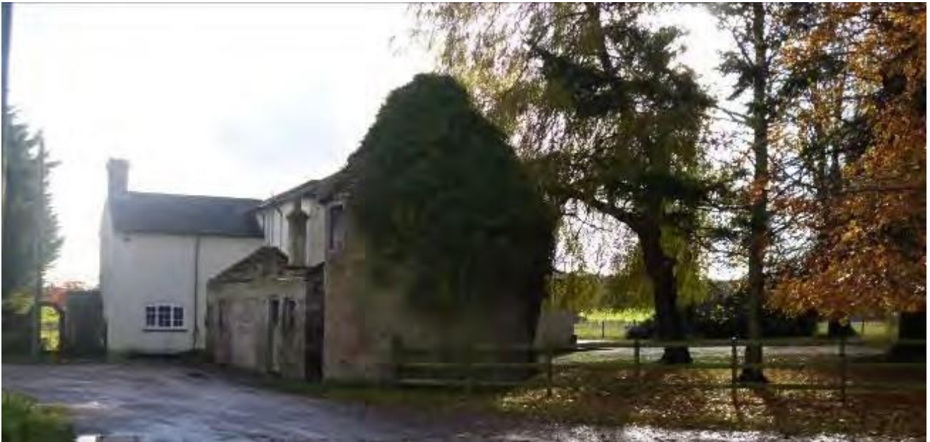
Plate 17: Oast-house at Barrow Hill Farm.
