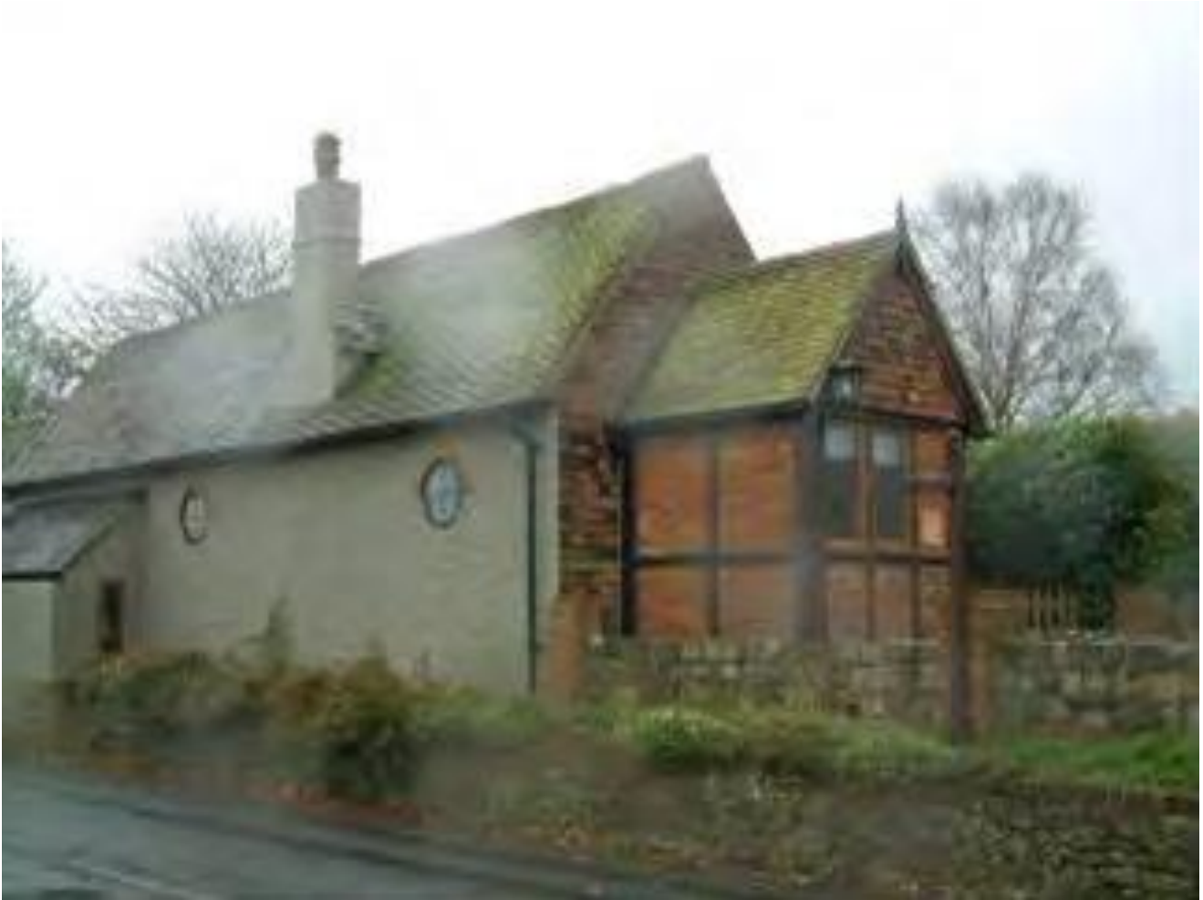
Plate 31: Example of potential medieval or early post-medieval building at Aldington Road
