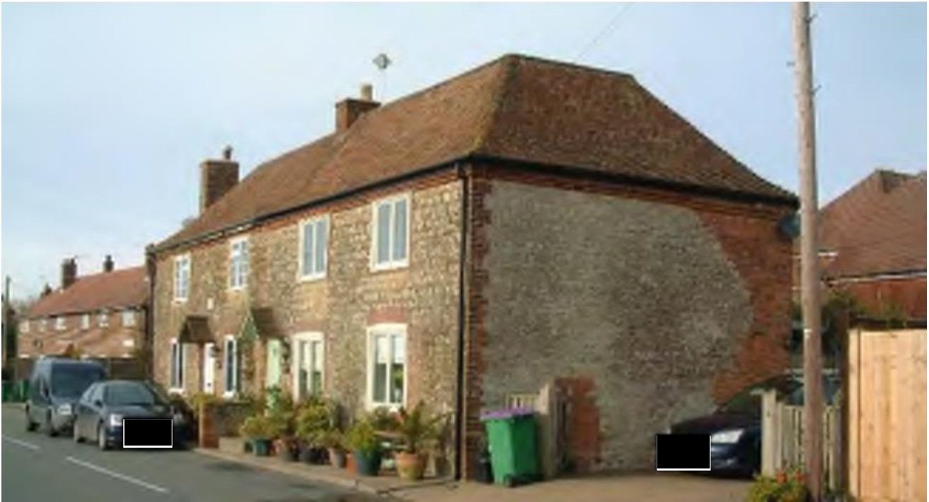
Plate 28: Forge Cottage viewed from the Aldington Road.
