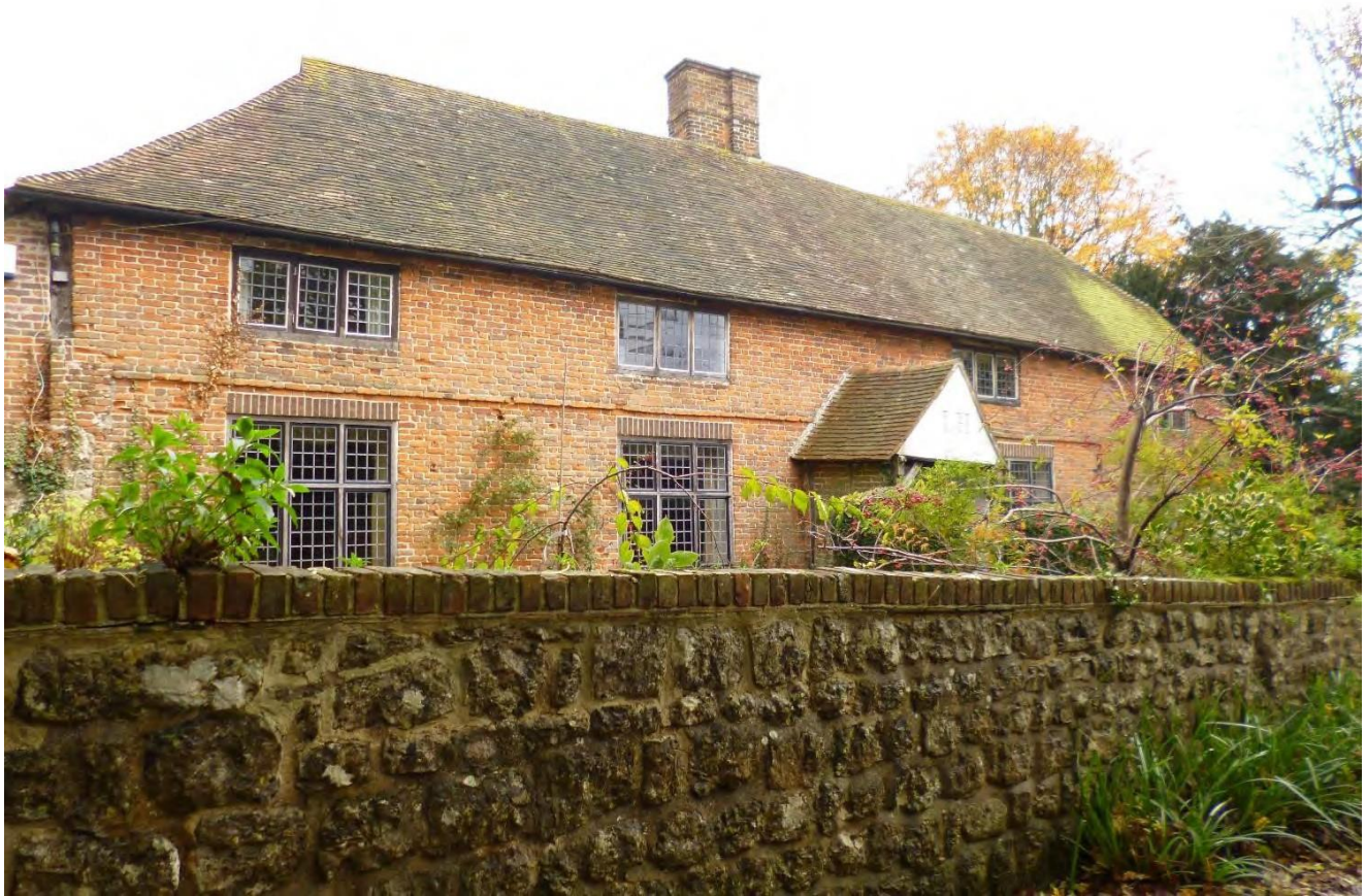
Plate 22: Lympne Hall (LB30) at centre of Lympne Conservation Area (view south east)
