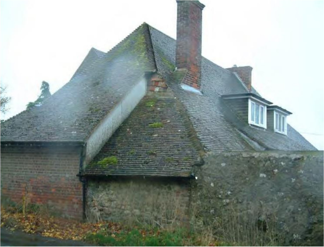
Plate 30: Example of potential medieval or early post-medieval building at Aldington Road
