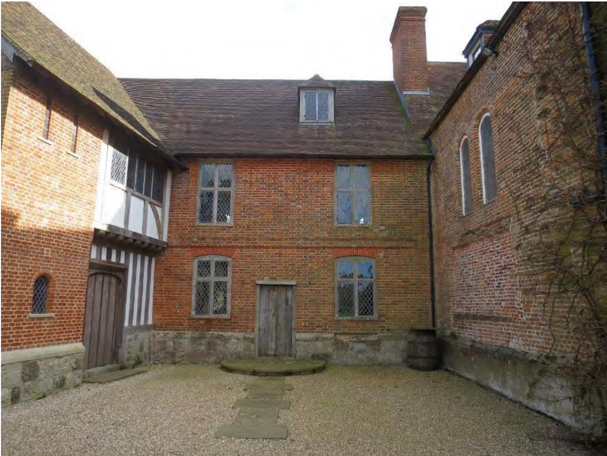
Plate 11: Open courtyard of the Manor House, view east
