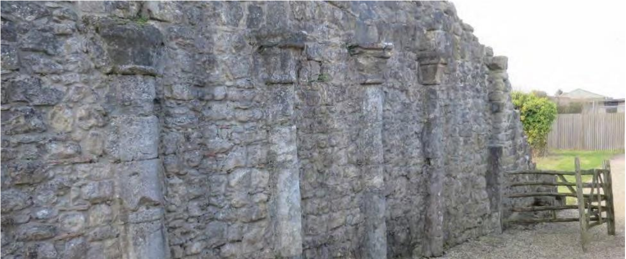
Plate 19: Pilasters at entrance to gatehouse, view south-west
