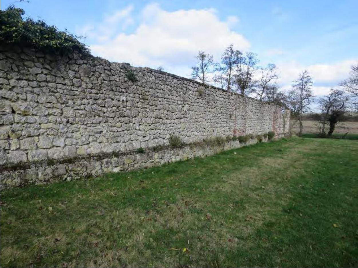
Plate 21: Perimeter wall to outbuildings (barns)
