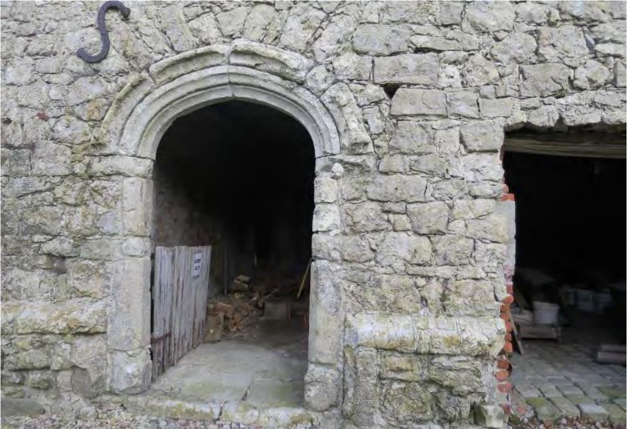
Plate 24: Moulded door surround one of two in south façade of east-west barn
