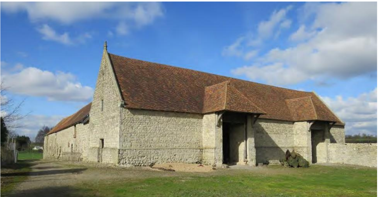
Plate 20: Grade I Listed north-south range of barns, view south-west
