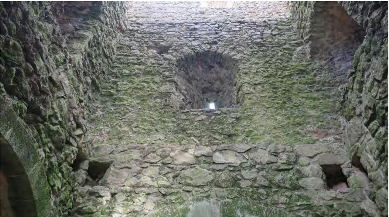
Plate 13: Interior of Rosamund's Tower, showing signs of water-ingress
