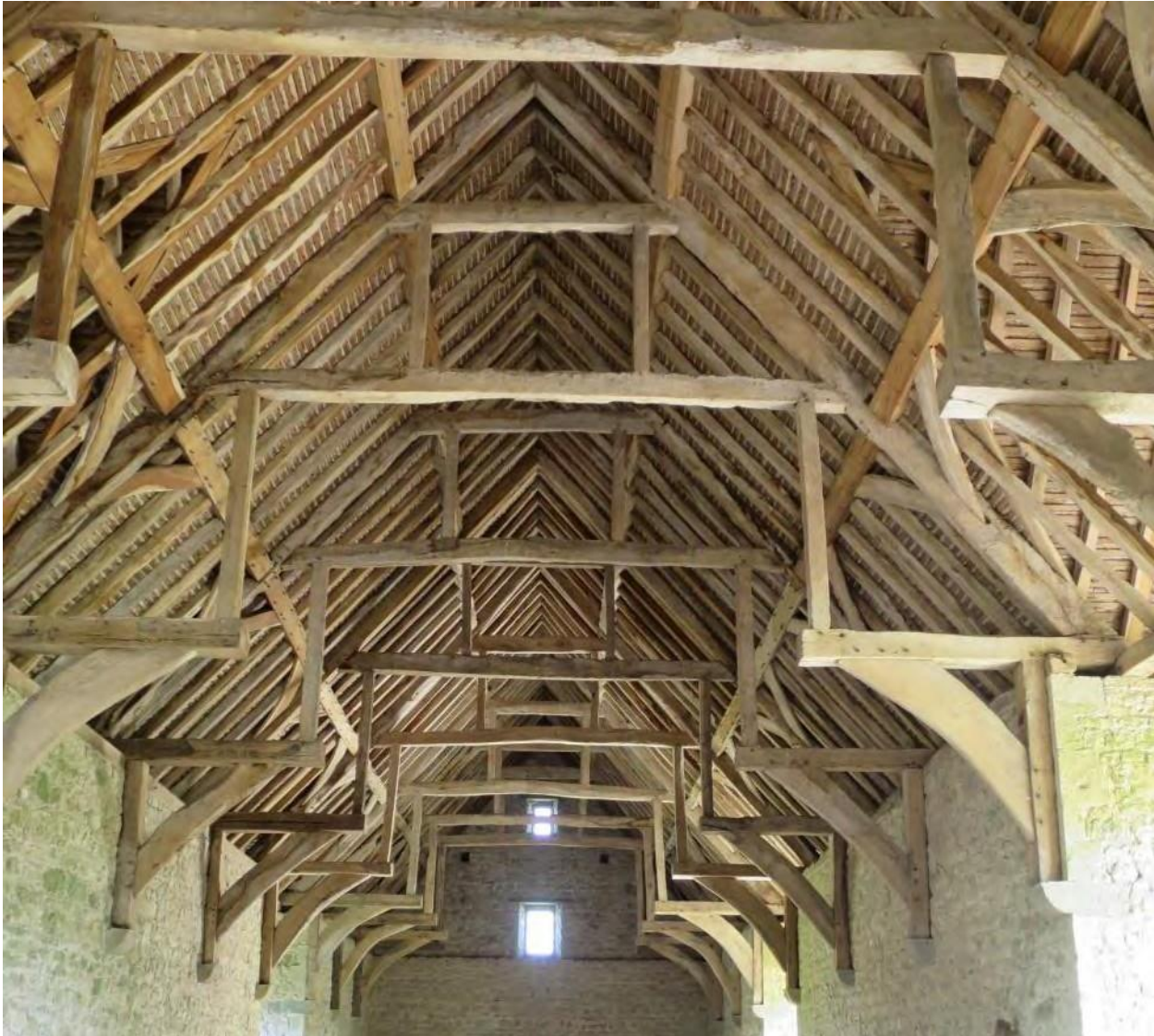
Plate 22: The north-south range of barns with hammer-beam roof
