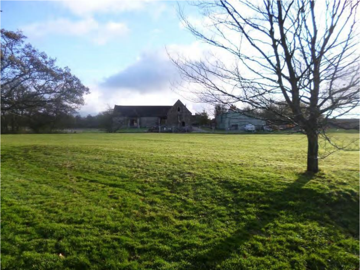
Plate 38: View east from near Farm Cottage towards the listed barns
