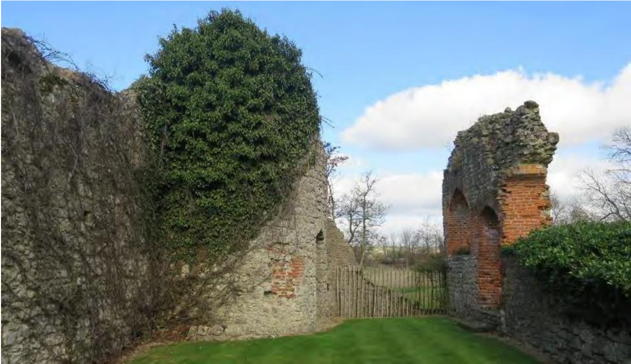
Plate 16: The former chapel and north-west tower view north
