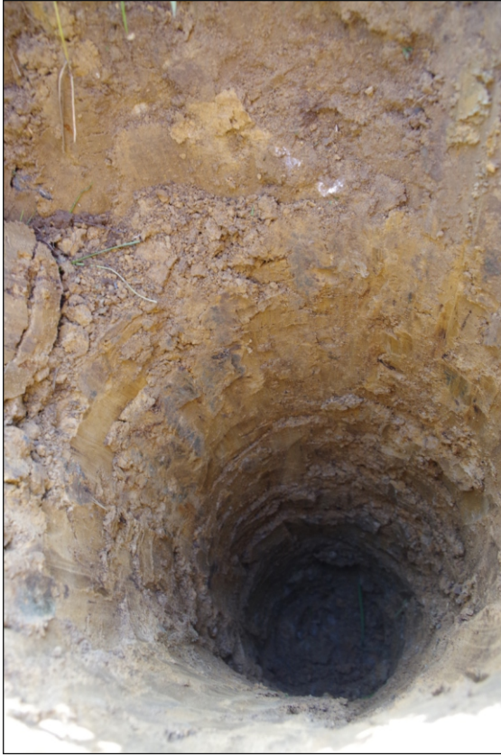
Plate 3: Borehole BH207 at 1.2m below ground level
