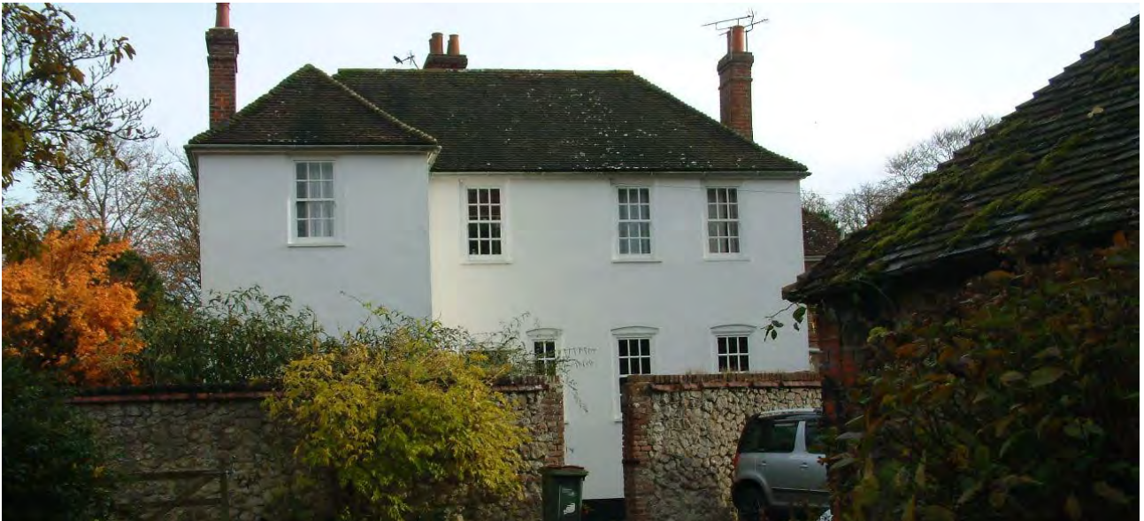
Plate 40: The Farmhouse at Belle Vue
