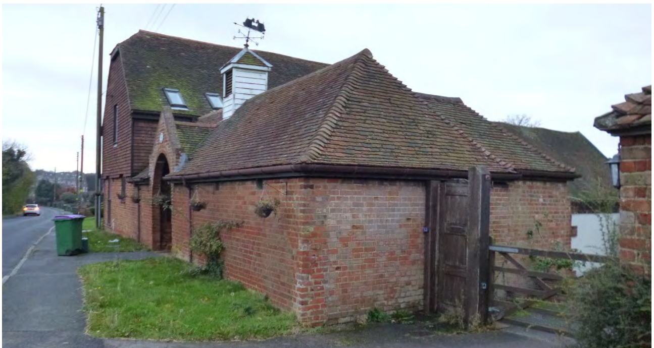
Plate 39: The South range at Newingreen Farm
