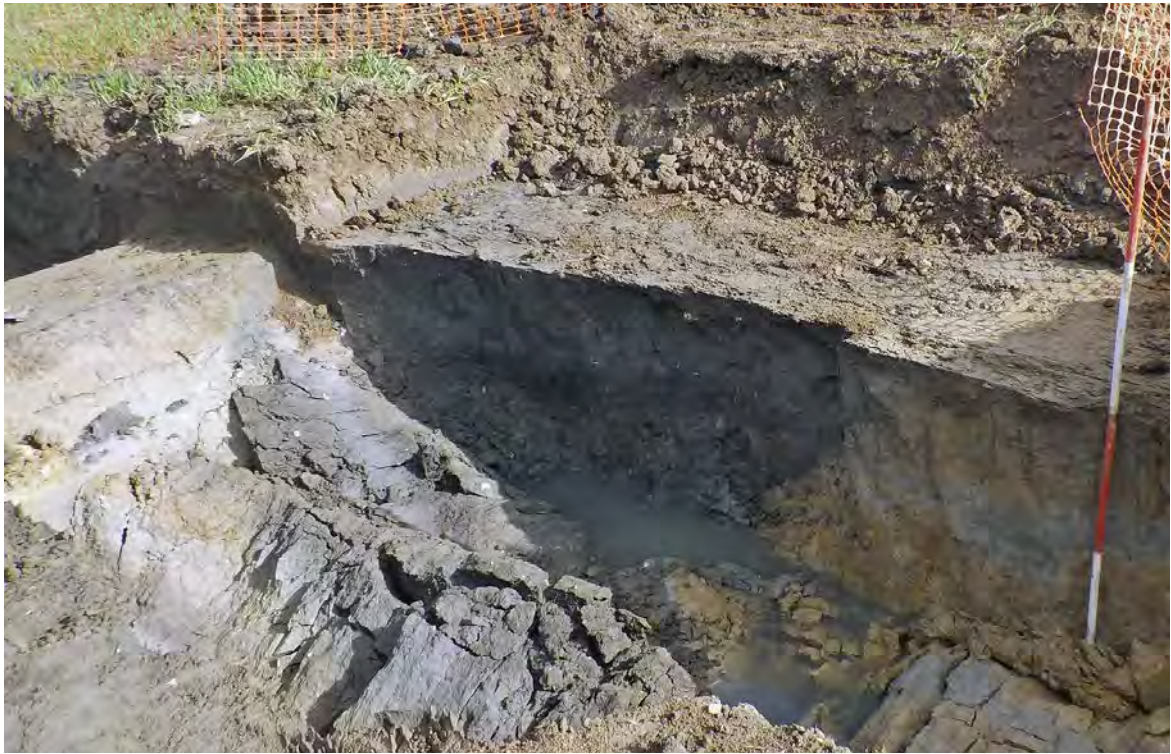
Plate 21: Ditch 25110 (after collapse), looking south-east
