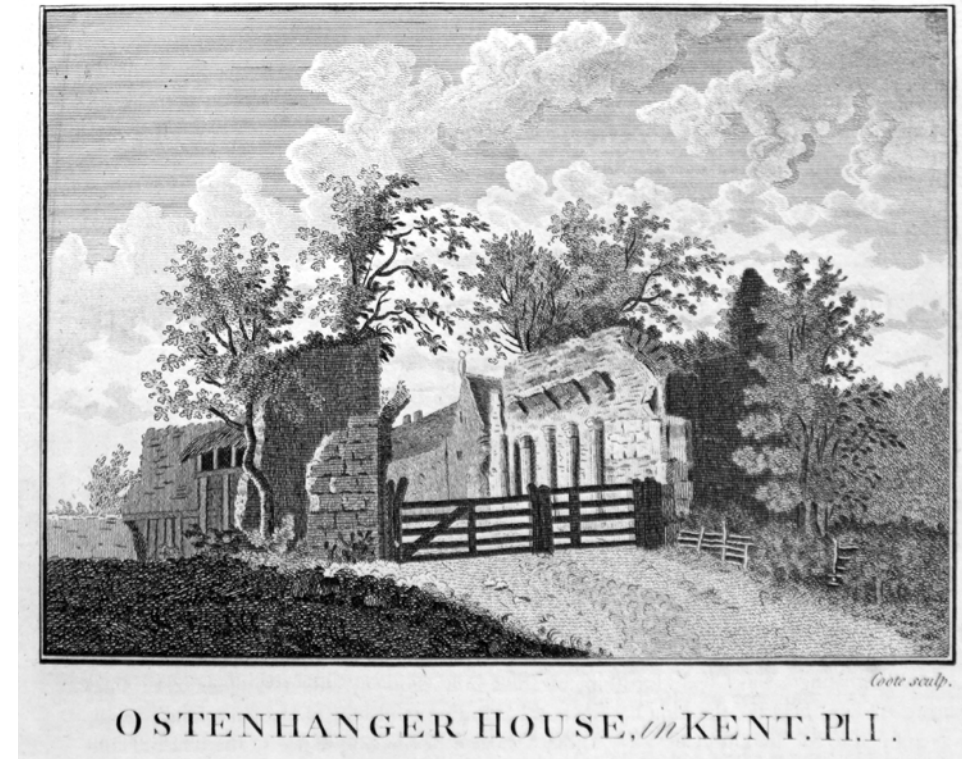
Figure 147: View looking west of the remains of the vaulted arch entrance to the gatehouse showing the barns in the background, from a sketch c.1750 or 1780 (British Library, reproduced in Archaeologia Cantiana Vol 31, 1915)
