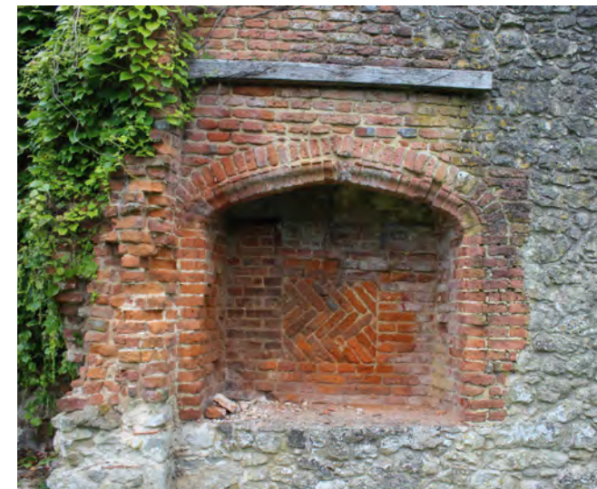
Figure 140: Red brick Tudor fireplace in the west range
