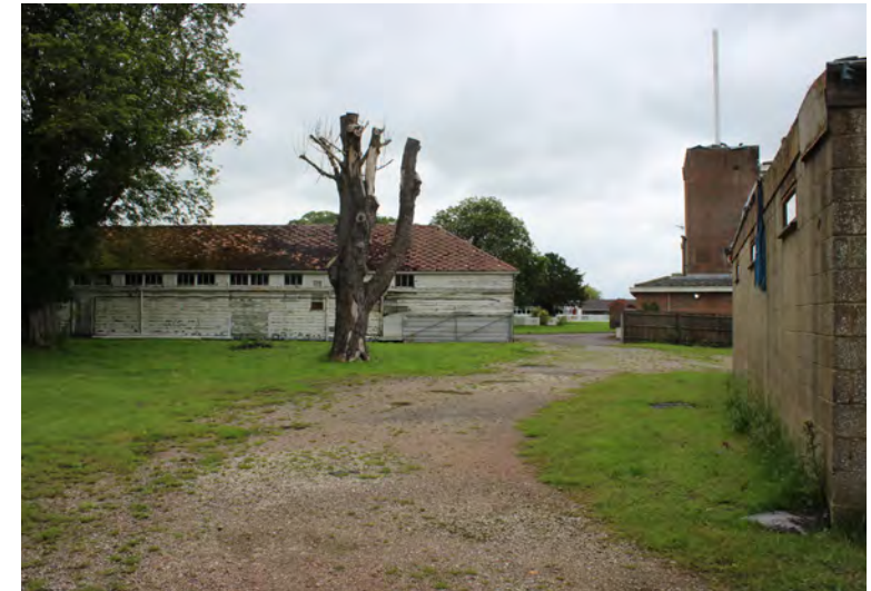
Figure 132: Former racecourse buildings to the east of the scheduled area
