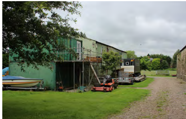
Figure 118: Modern stables and semi-permanent buildings to the south of east-west barn
