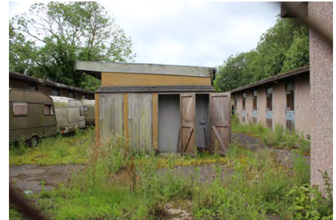
Figure 119: Modern stabling to the south of the barns
