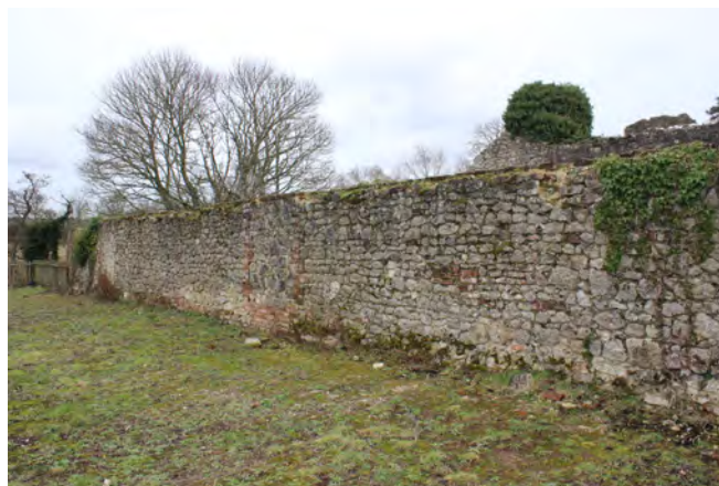
Figure 115: Detail of stone wall bounding the east side of the area to the east of the barns showing evidence of infilled openings
