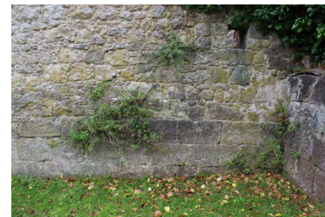
Figure 136: Early dressed ragstone ashlar blocks, found at the lower courses of the curtain wall near the base of the gatehouse, which pre-date the 14th century
