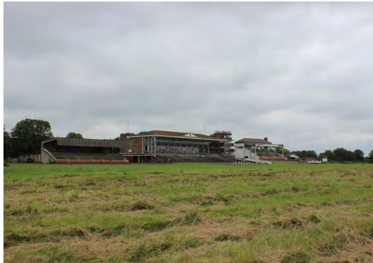
Figure 131: Former racecourse grandstands to the east of the scheduled area
