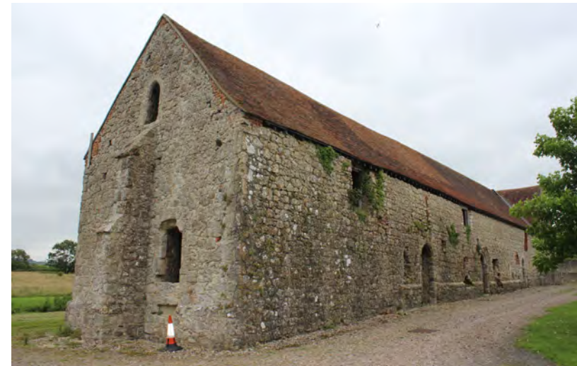
Figure 84: View of the west gable end and south elevation looking north-east
