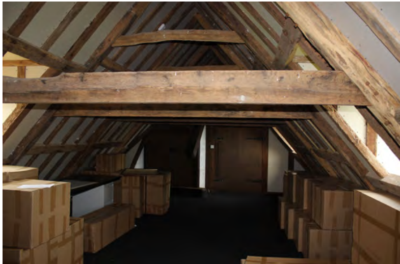
Figure 70: Loft storage space in the main range
