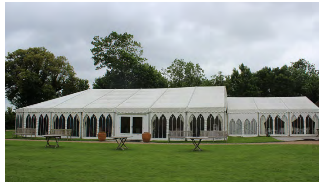
Figure 82: View looking south across Inner Court towards the temporary marquee structure
