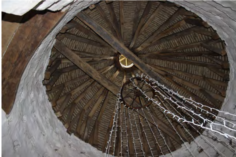
Figure 69: Conical timber roof to the north-east tower
