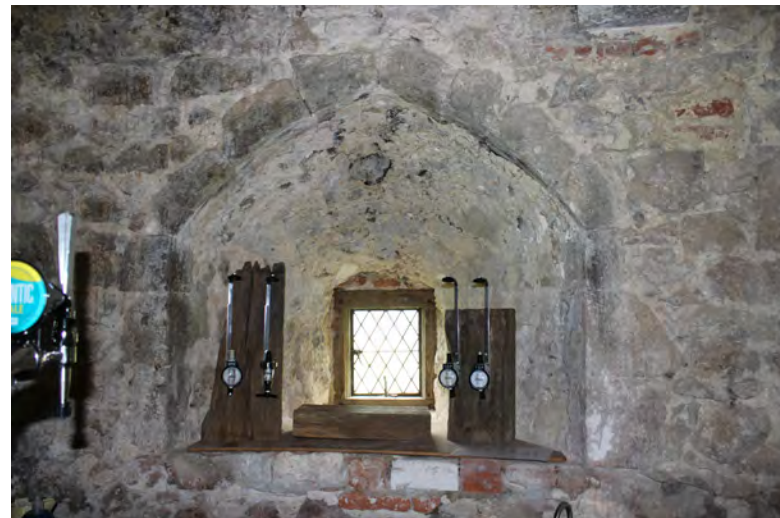
Figure 68: Modified window in north-east tower
