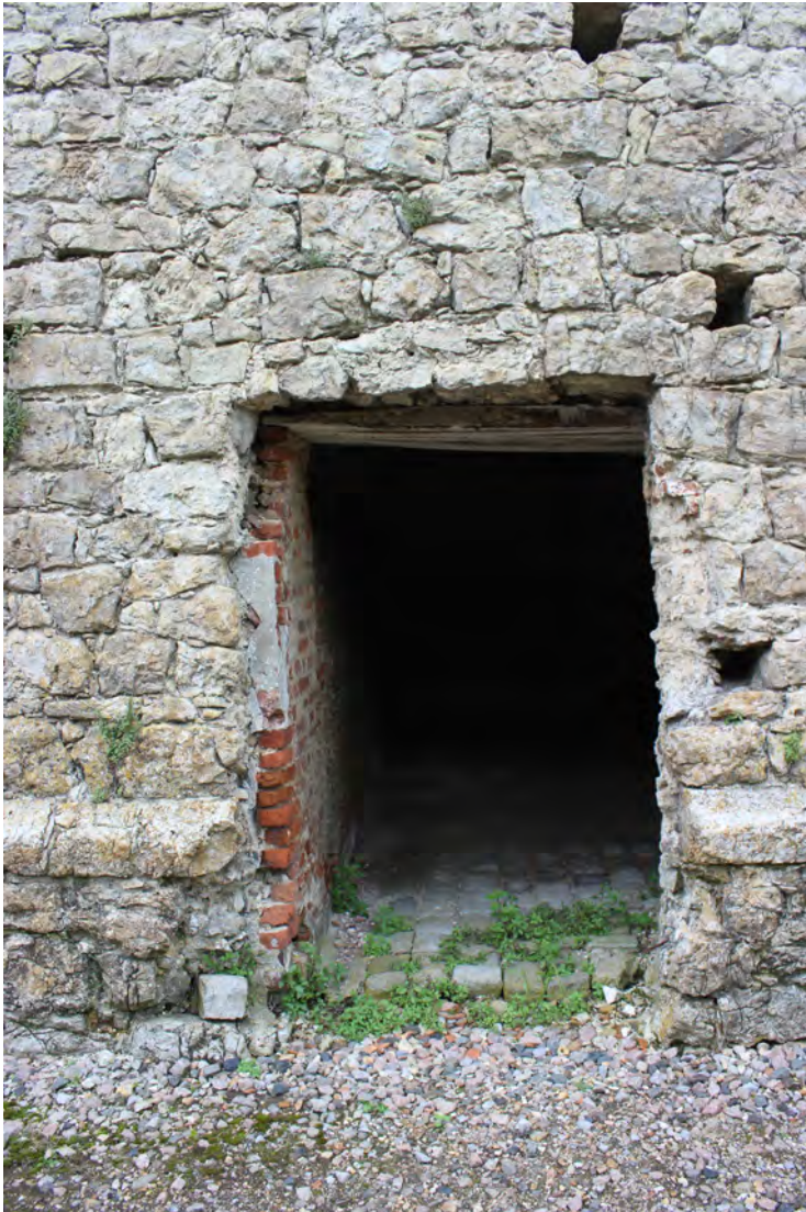
Figure 86: Later inserted doorway featuring a flat arch and later brickwork
