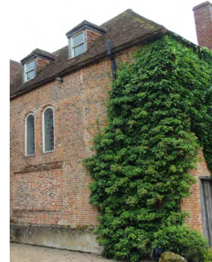
Figure 42: View of the main range showing the north elevation which features 16th century elements
