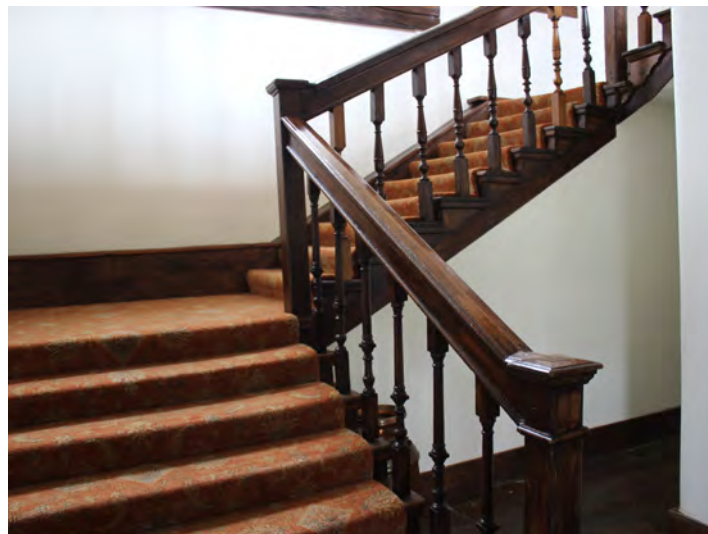
Figure 54: Historic staircase, potentially including 16th century fabric
