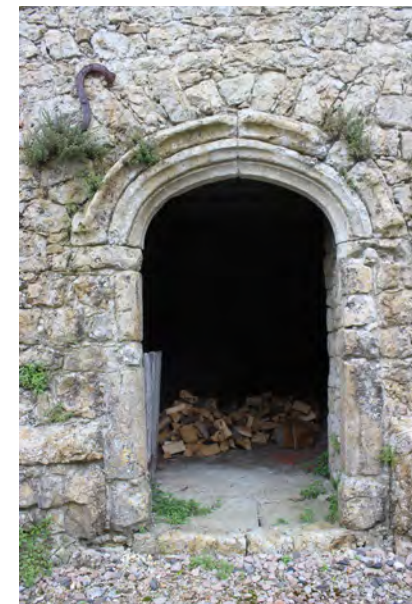
Figure 89: Historic doorway with moulded surround and a hood mould
