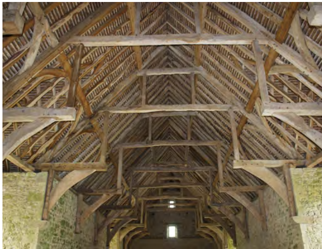
Figure 110: Detail of the hammerbeam roof structure
