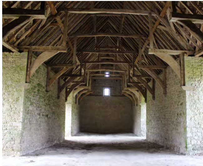
Figure 108: View looking north towards the north internal elevation
