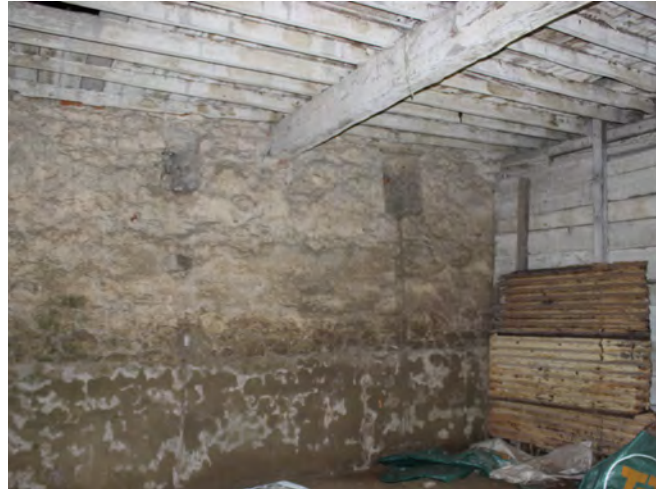
Figure 95: View of the room to the east of the central room showing a timber partition to the east and a timber joist floor above
