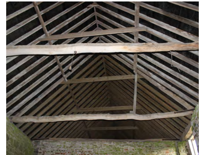
Figure 93: Roof structure in the west room showing largely modern timbers
