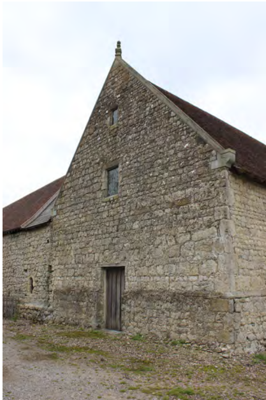
Figure 105: View of the south gable looking north-west showing the original window openings and the later doorway below
