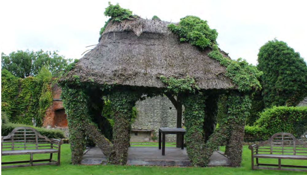
Figure 83: View of the wedding pavilion looking west
