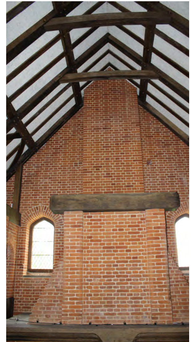
Figure 74: Pitched roof and gable detail to modern extension
