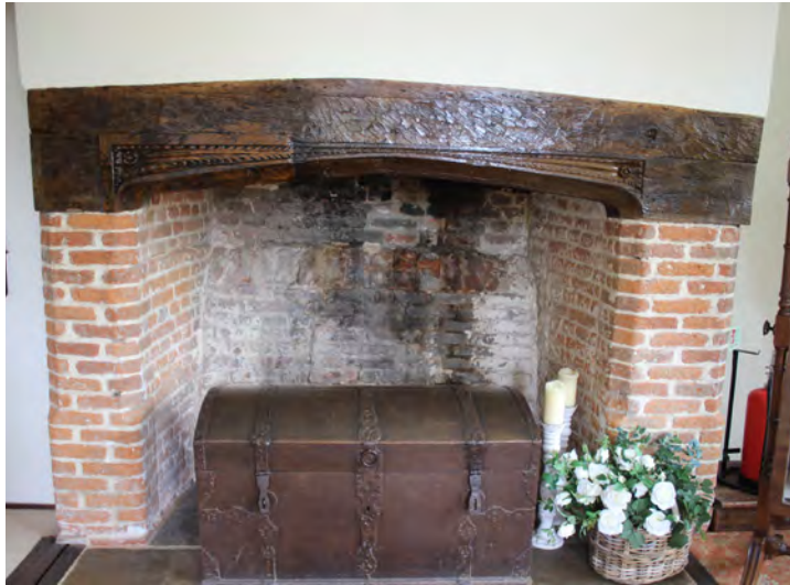
Figure 56: 15th century chamfered brick fireplace with arched wooden bressummer and carved spandrels at first floor
