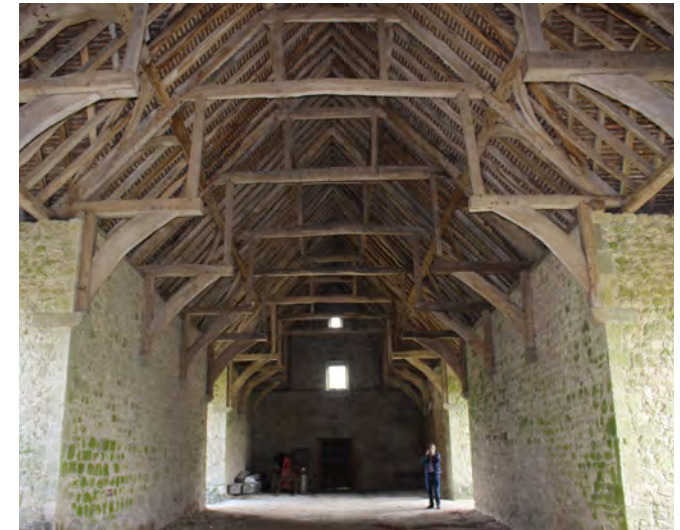
Figure 109: View looking south towards the south internal elevation
