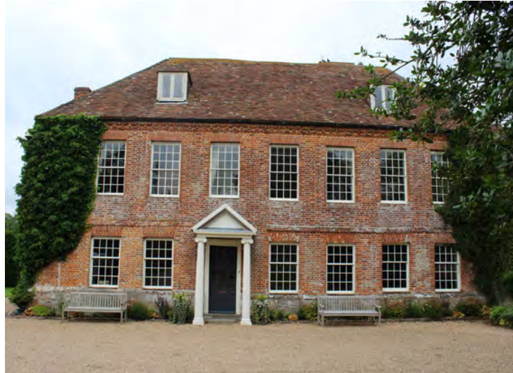
Figure 41: View of the main range showing the south-facing, Georgian frontage with an unbalanced composition of bays
