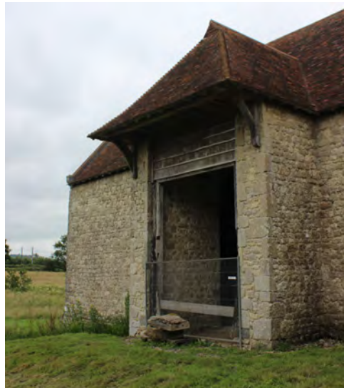
Figure 103: View of a representative wagon porch
