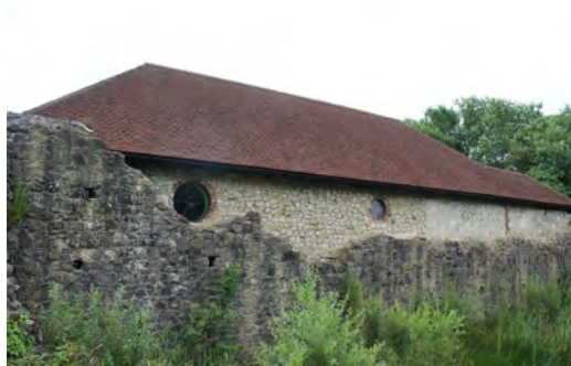
Figure 80: View from the east entrance to the castle complex showing the modern services building abutting the southern section of the west curtain wall
