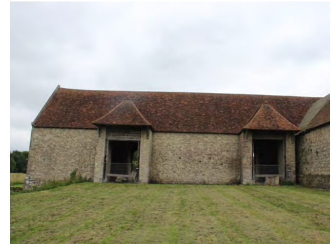
Figure 102: View of the west elevation looking east showing two wagon porches and the adjoining east-west barn on the right
