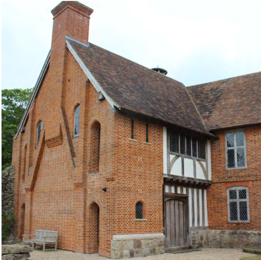
Figure 50: View of the modern north range
