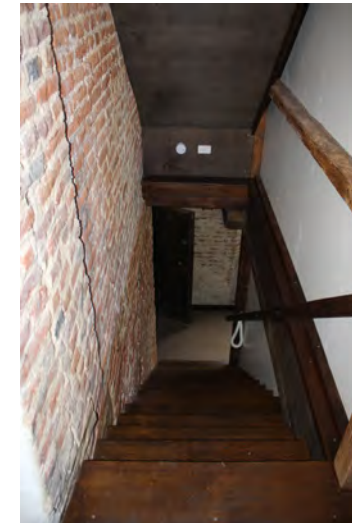
Figure 62: Modern stair accessing the upper level of the rear wing
