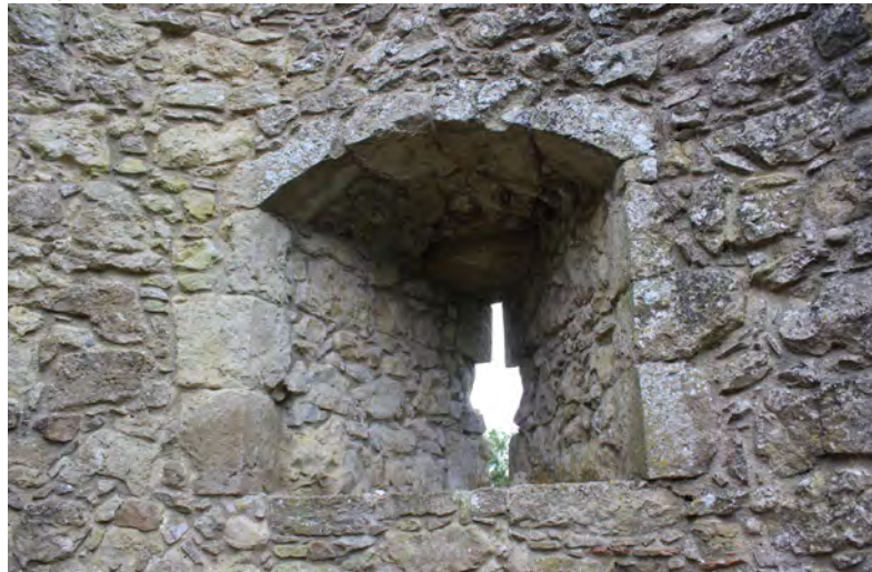
Figure 30: View of an arrow slit window in the north-west tower
