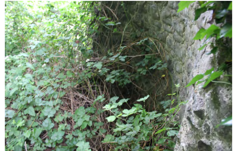
Figure 33: View of the internal wall of the south-west tower looking north-west
