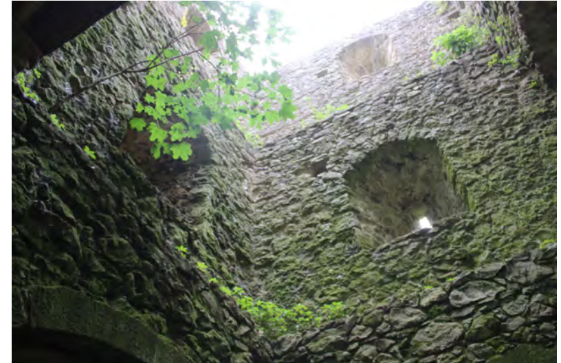
Figure 37: Internal view inside Rosamund's tower showing three distinct levels
