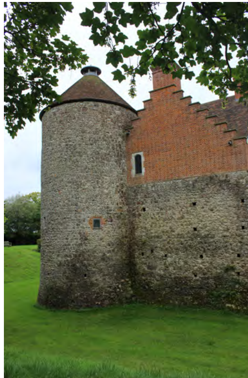
Figure 25: View of the north-east tower looking south
