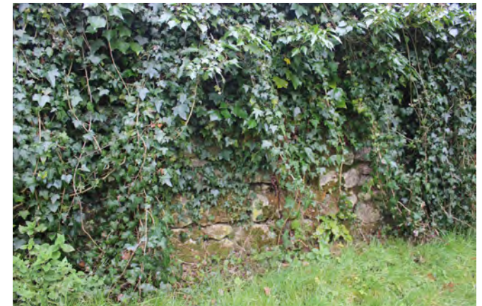
Figure 12: Detail of bridge showing stone materiality beneath the ivy
