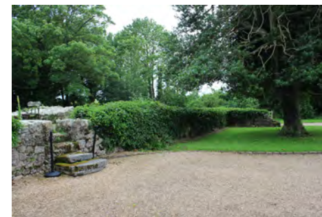
Figure 18: View looking south-east from the Manor House showing the lower remains of the east curtain wall to the south of the bridge entrance and the lower remains of the main range from the Manor House
