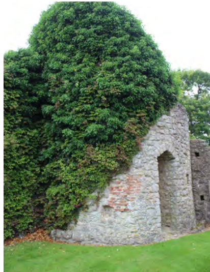
Figure 28: View of the north-west tower from Inner Court looking north
