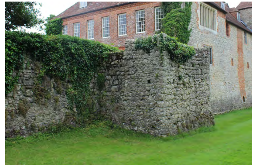
Figure 27: View of the south-east tower looking north-east
