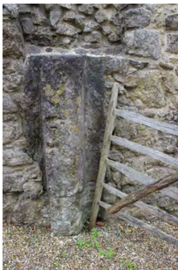
Figure 05: Groove for the portcullis in the gatehouse entrance
