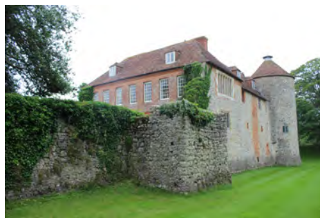
Figure 17: View of the east curtain wall looking north-west showing the north section and the north-east tower incorporated into the Manor House and the lower remains to the south. The east arm of the moat is dry.
