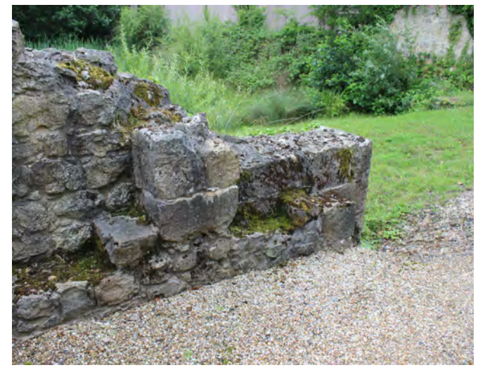
Figure 09: Pivot hole for the former drawbridge in the gatehouse entrance
