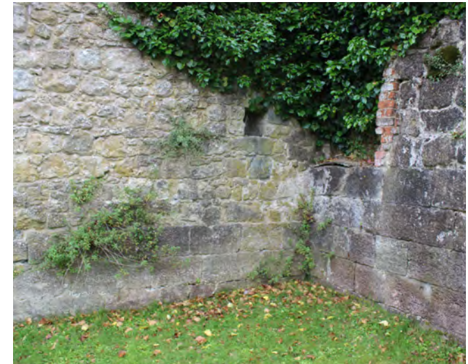
Figure 08: Detail of the lower courses of ashlar or cut blockwork which may indicate an earlier phase in the castle's construction
