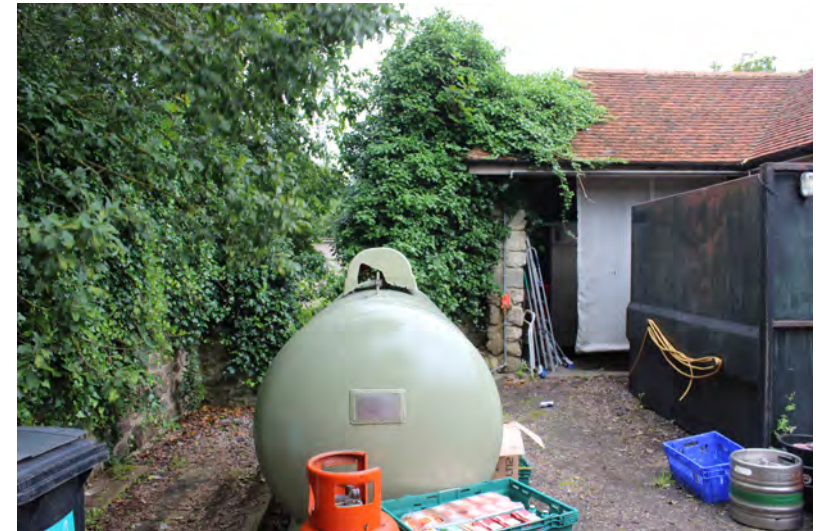
Figure 34: View looking towards the south-west tower, which is obstructed by modern plant relating to the services building
