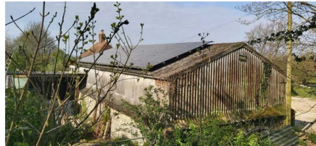
Old Barn with PV panels and interesting plinth detail
