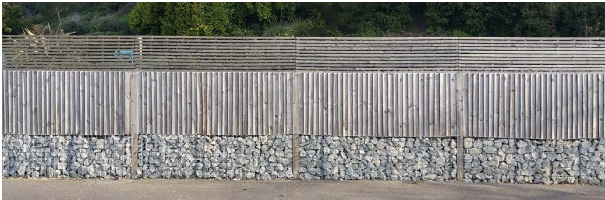
Garden fence in Sandgate : weathered timber with gabion wall base. Subdued colours and interesting detailing.
