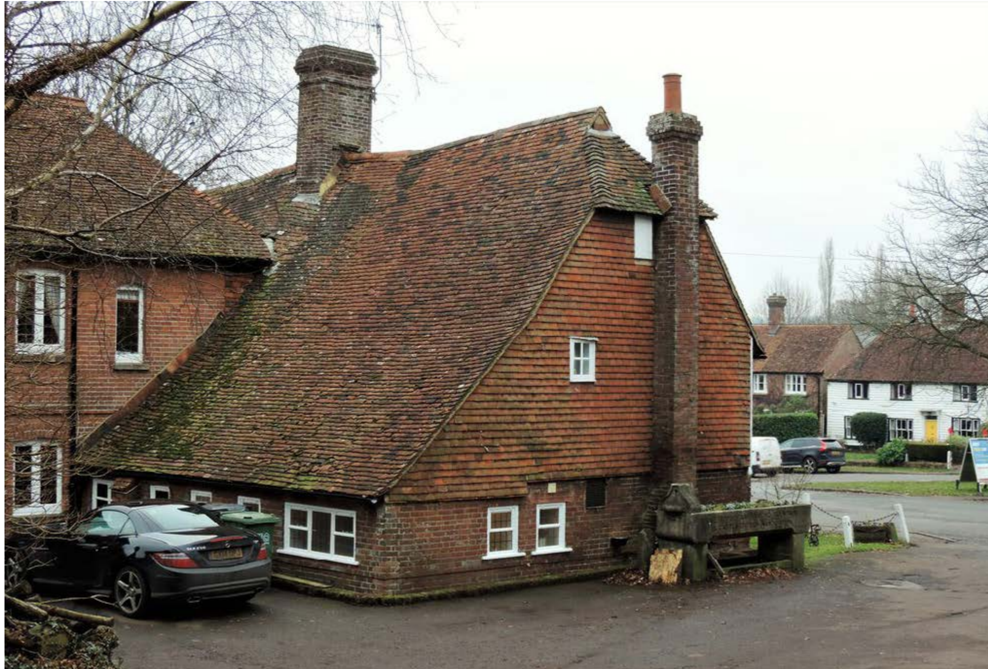
Note the very low eaves line at the rear of the catslide
