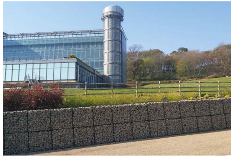
Gabion Walls : open rock and metal baskets are used quite frequently in the area and are very appropriate, contemporary details.
