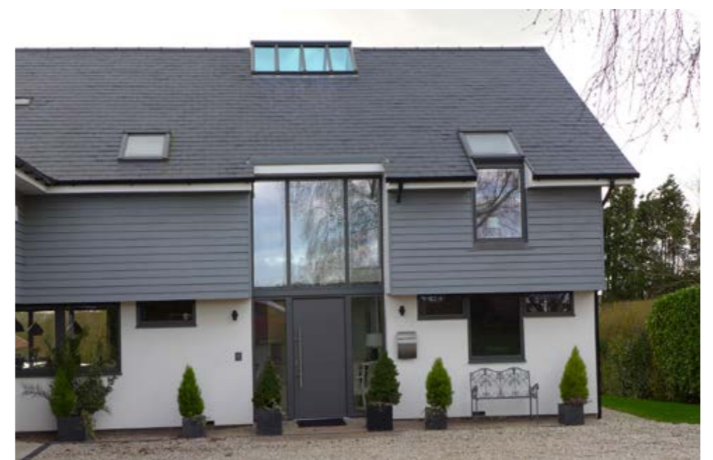
A modern home on Stone Street, using many traditional vernacular details and a neutral grey colour scheme. Care needs to be taken regarding the uniform nature of contemporary materials in relation to context.
