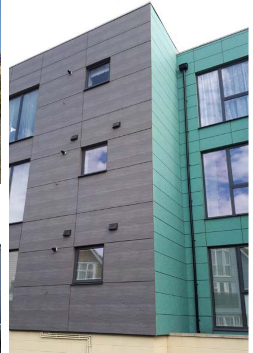
Detail Above demonstrates glossy modern facade materials which are not relevant to the area. This image also highlights the need for very careful detailing of panels, joints and corners when experimenting with new materials.
