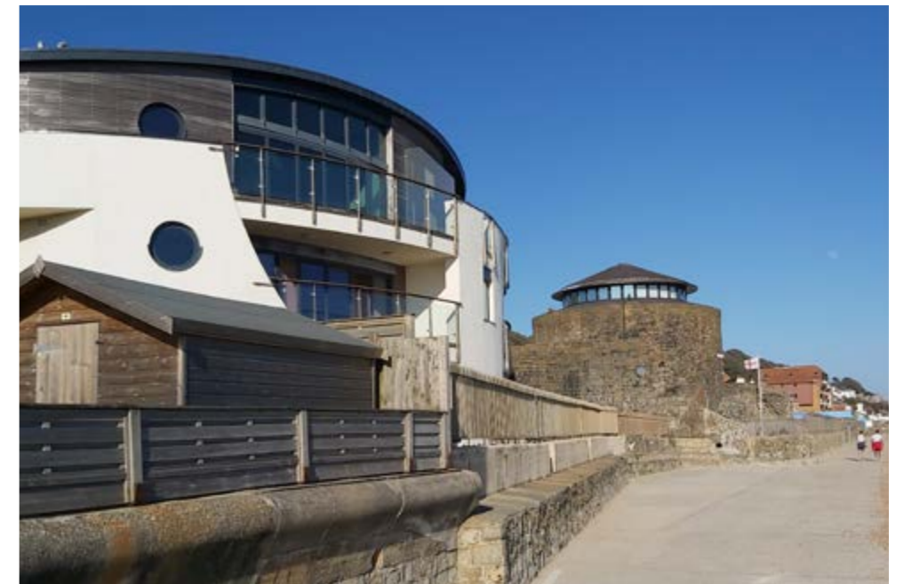
SAGA office by Michael Hopkins, a high-tech glass and steel structure sitting in comfortable contrast to the finely grained historic town below it.
