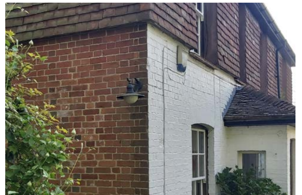
A really nice example of tile hanging above, with brickwork plinth and a change in material / paint colour at the corner.
