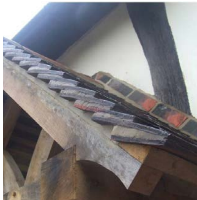
Multiple pitches, gable and hipped ends, bays and dormers along with very bold vertical chimney elements contribute to a diverse skyline. Note the elegant, exposed tile edge detail.
