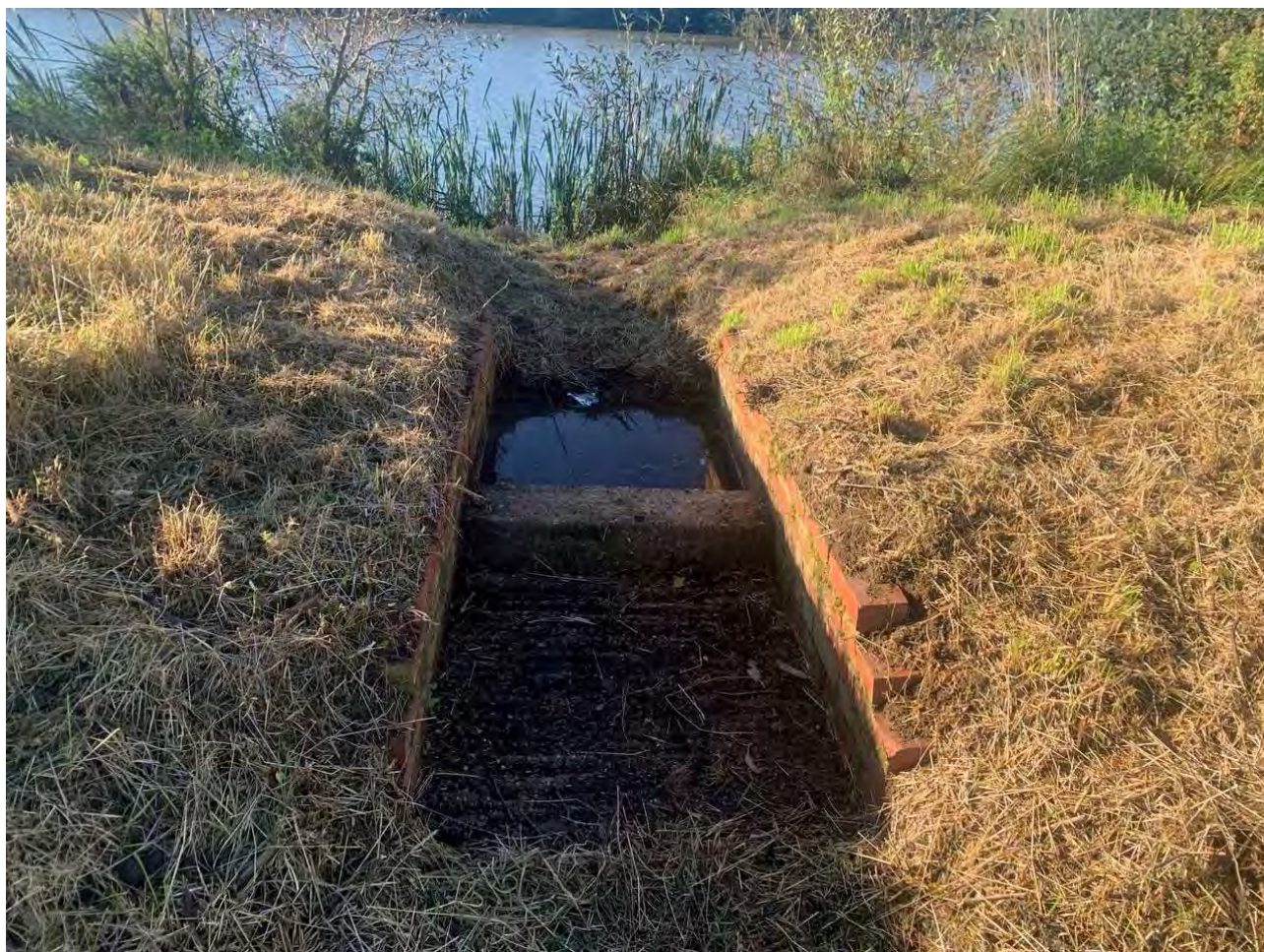
Figure 29 Existing spillway at the northern bund of the racecourse lake
