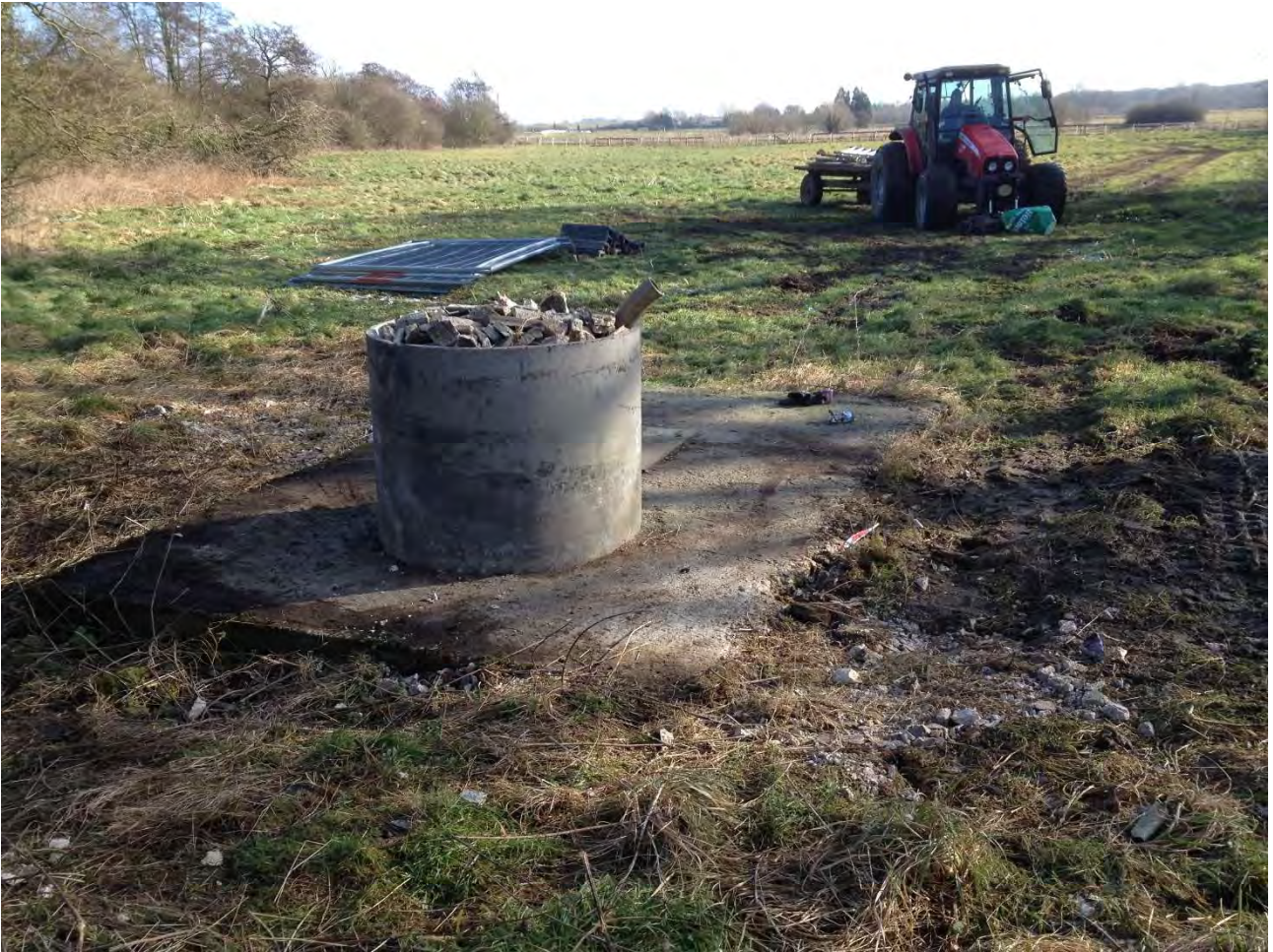
Figure 30 Decommissioned former pumping site at the western edge of the racecourse lake
