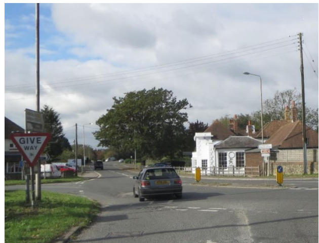
Figure 14 Hythe Road approaching Newingreen junction
