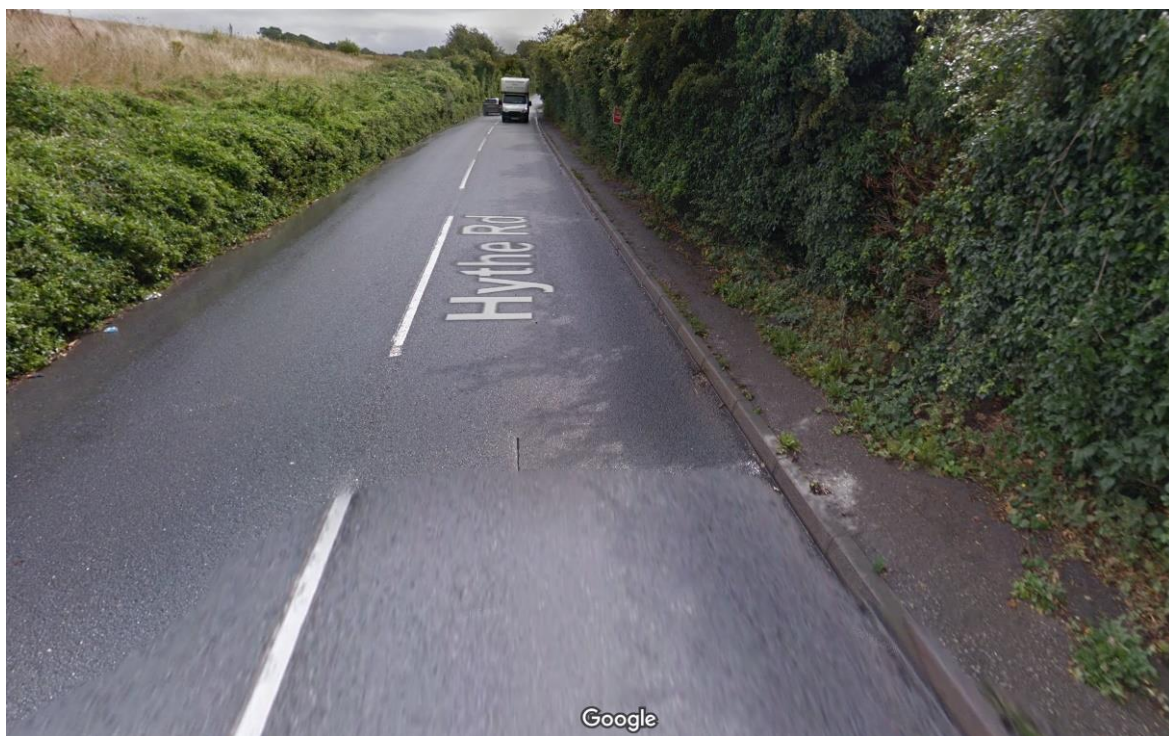
Photograph 10 Narrow footway along southern side of A261 Hythe Road to the east of the junction with Aldington Road
