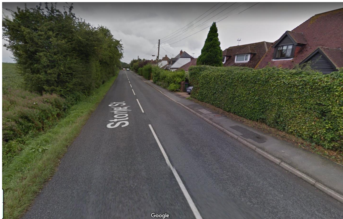
Photograph 7 Footway along one side of Stone Street, south of junction with A20 and A261
