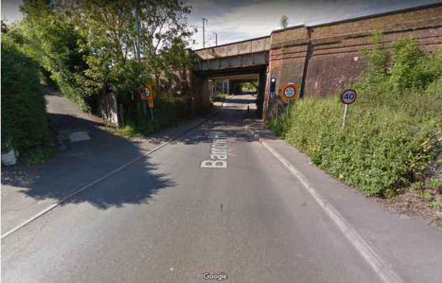
Photograph 5 Footway along both sides of A20 under rail bridge towards Sellindge
