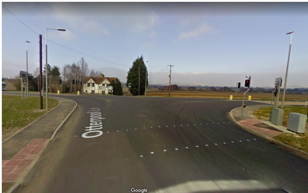
Photograph 6 Pedestrian crossing facilities at A20/Otterpool Lane signalised junction
