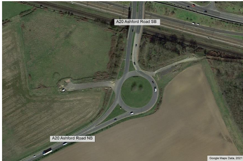
Figure 57 A20 Ashford Road small roundabout
