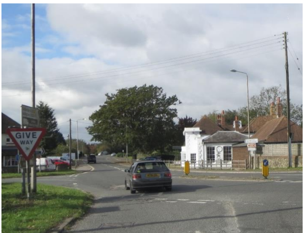
Photograph 8 Hythe Road approaching Newingreen junction
