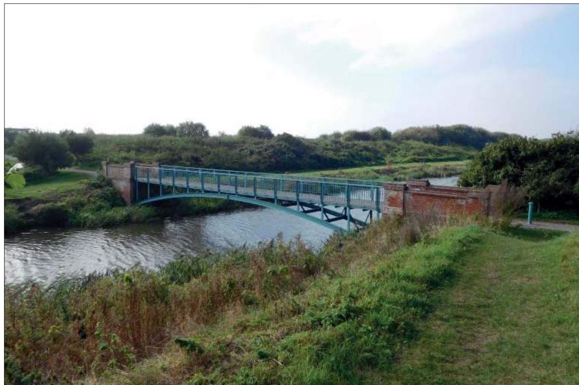
Photo 18: Illustrative view south-west across the Royal Military Canal from public bridleway HB65.
