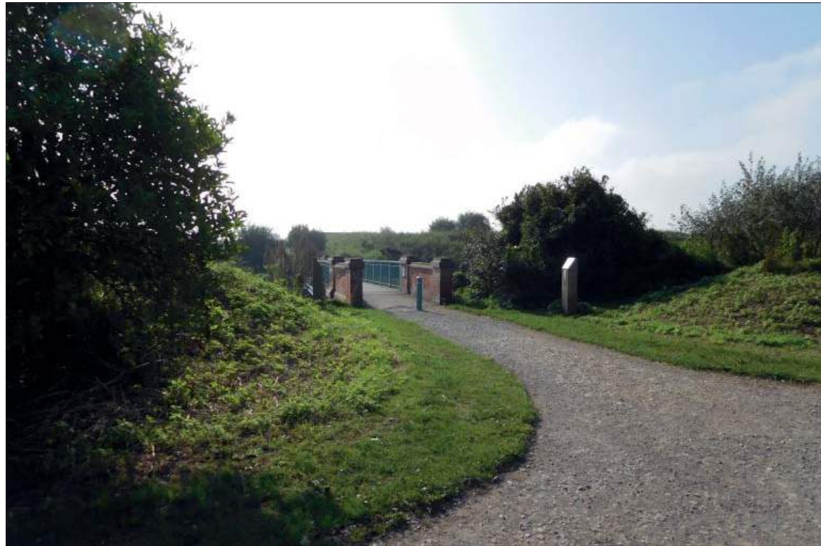
Photo 21: Illustrative view south towards the Royal Military Canal from public bridleway HB65.
