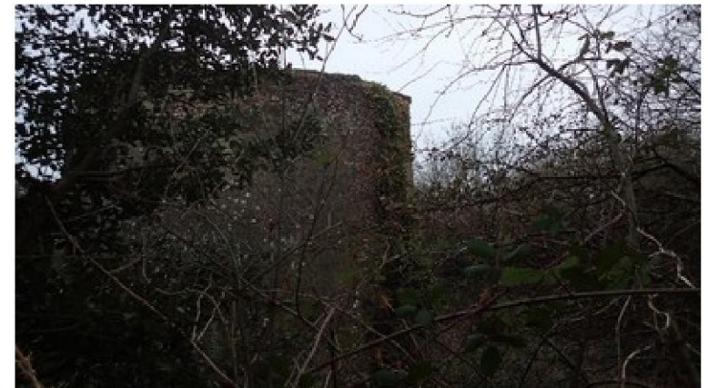
Martello Tower No. 9
