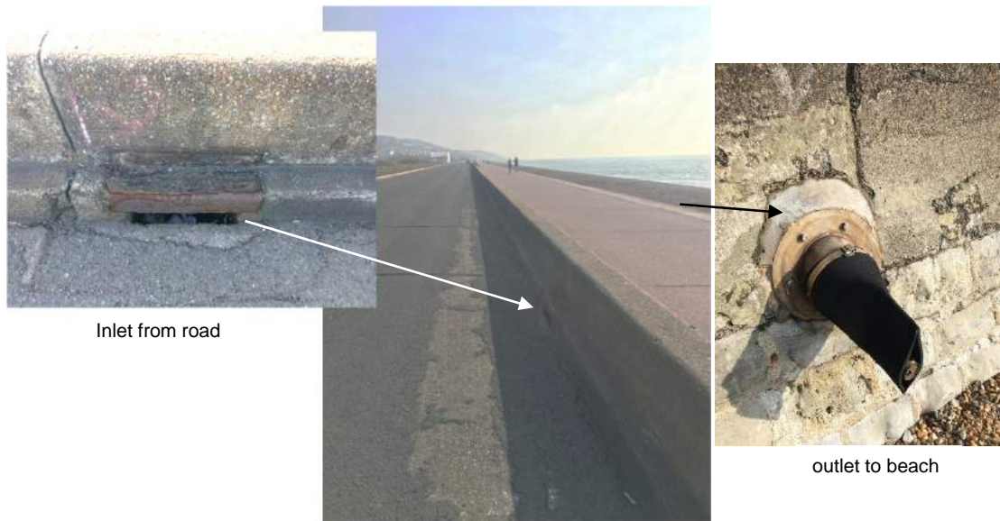
Figure 3.3 – Existing road drainage along Princes Parade.
