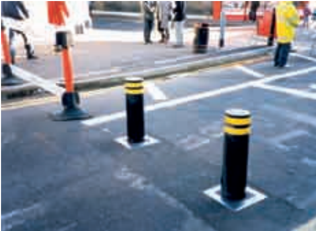
Fig. 3.7 Rising bollards raised and lowered
