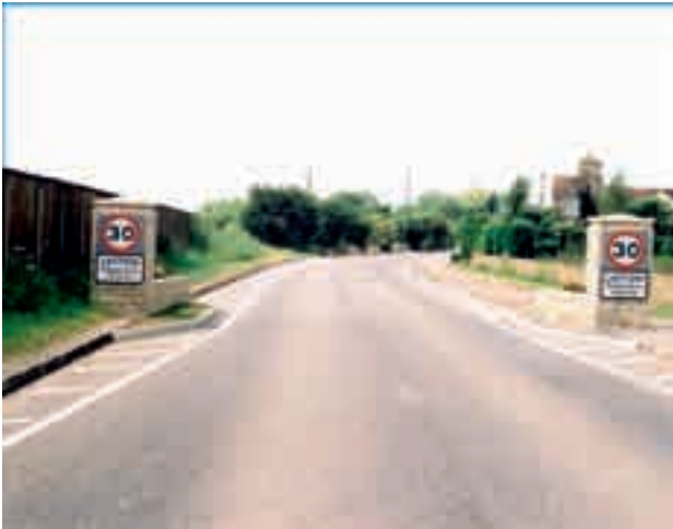
Fig. 3.8 Gateway feature, Latton
