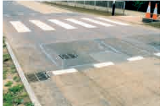
Fig. 4.8 'H' road humps
