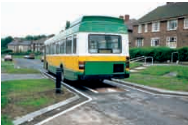
Fig. 4.14 Cushion and associated build-out (left) and cushion in narrowing
